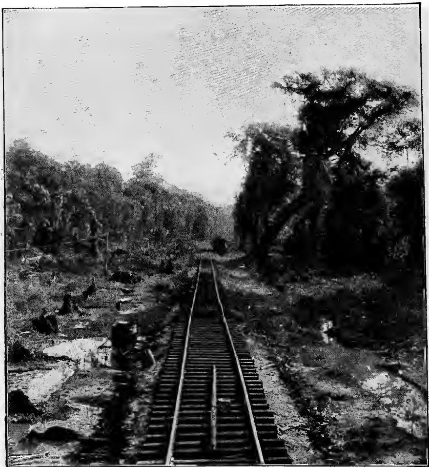
COMPLETED R. R. THROUGH SWAMP.
