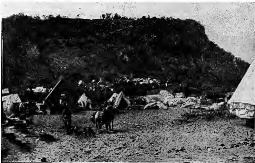
SIBONEY—CAMP OF ARMY ENGINEERS ENGAGED IN BUILDING A DOCK AND OPERATING THE SHORE RAILROAD.
