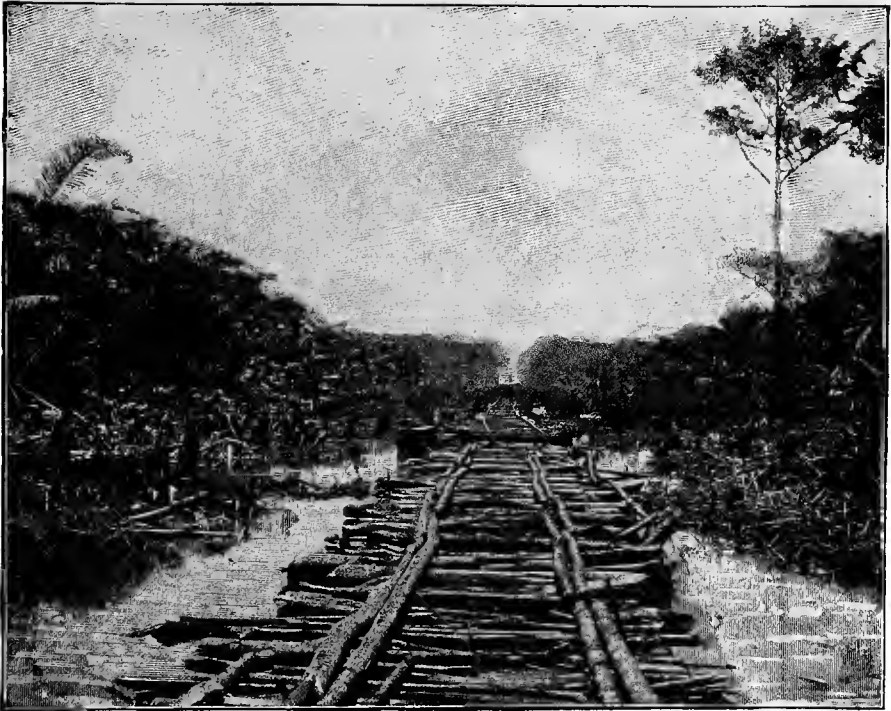
BUILDING R. R. THROUGH SWAMP.
