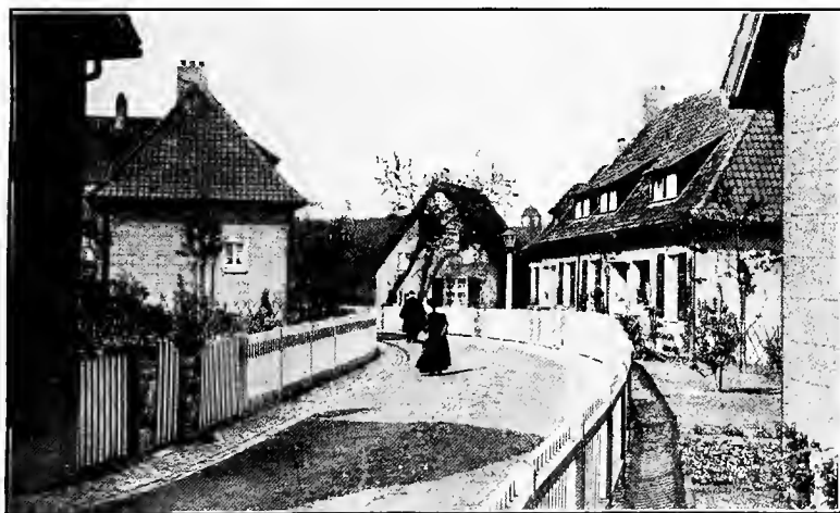
ATTRACTIVE AND INEXPENSIVE STREETS OF THE KRUPP WORKINGMEN'S COLONIES, NEAR ESSEN, GERMANY
