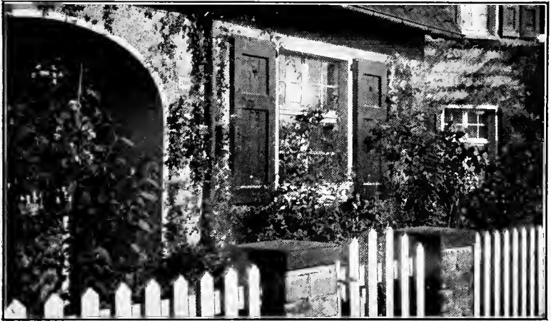
EXTRA SPACE FOR UNUSED ROAD LEAVES LITTLE SPACE FOR MUCH USED GARDEN—AN EXAMPLE FROM EUROPE
