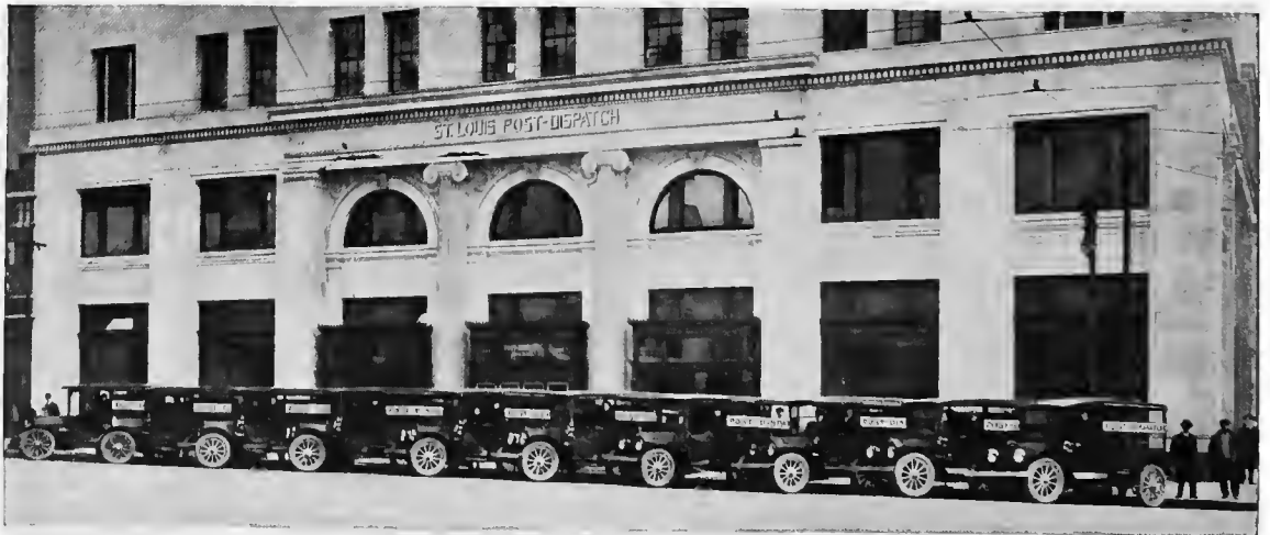
FLEET OF POST-DISPATCH DELIVERY TRUCKS
