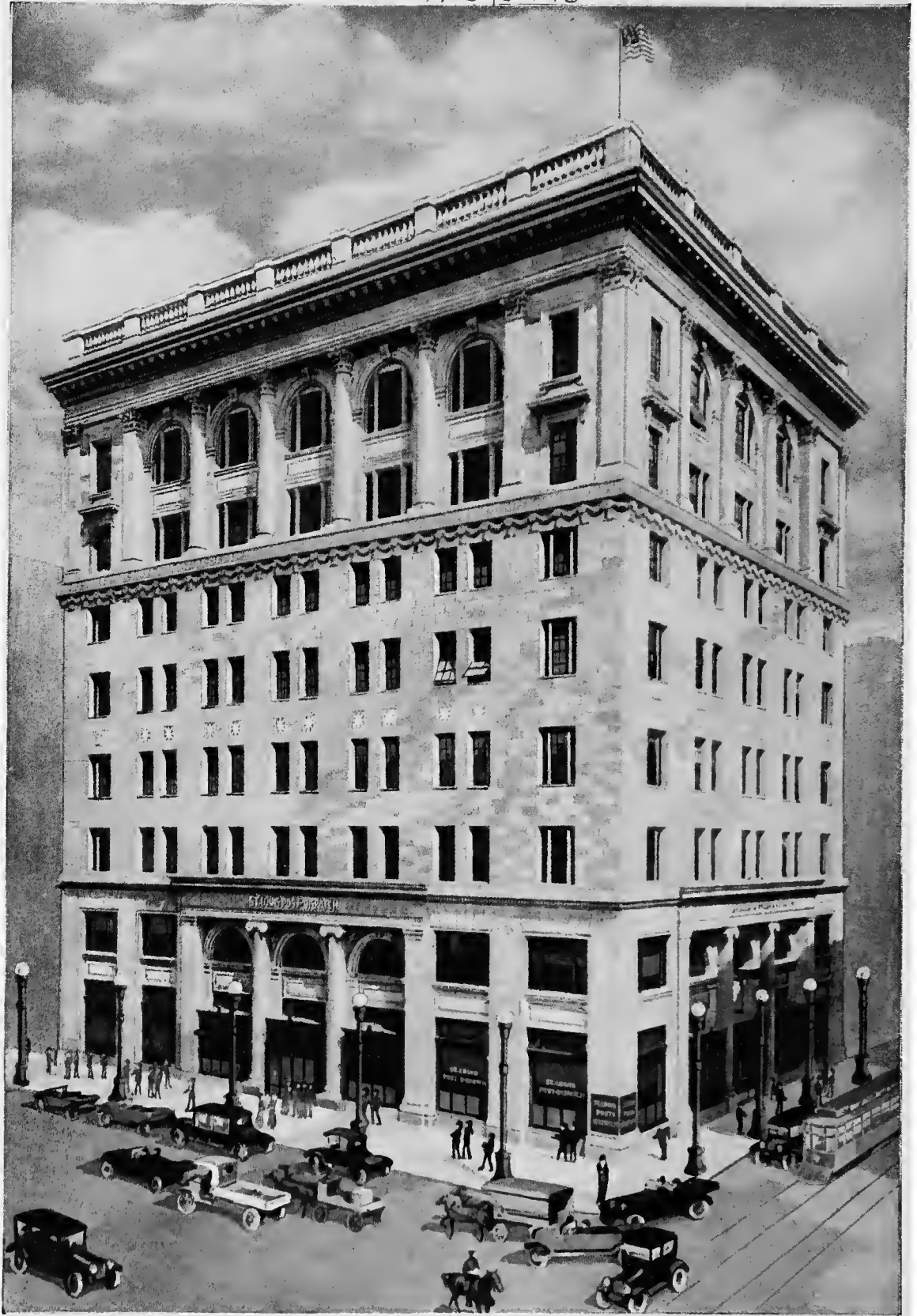
THE NEW POST-DISPATCH BUILDING, TWELFTH AND OLIVE STREETS, ST. LOUIS
