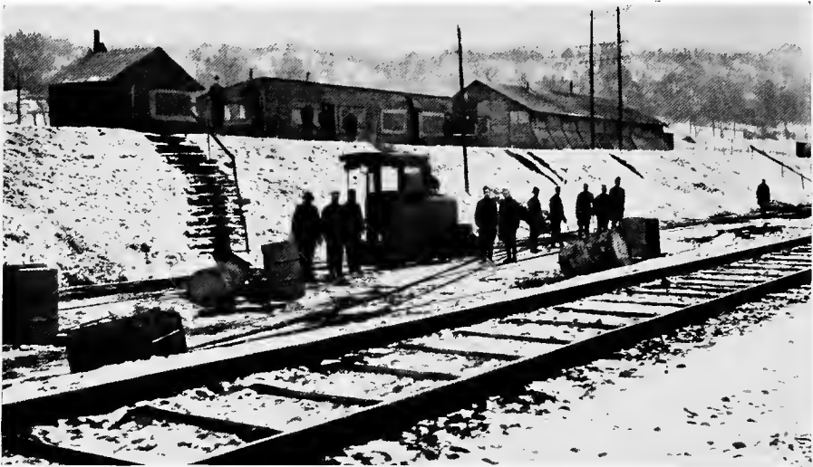
"F" COMPANY'S BARRACKS AT BELLEVILLE 35 H. P. TRACTOR IN FOREGROUND
