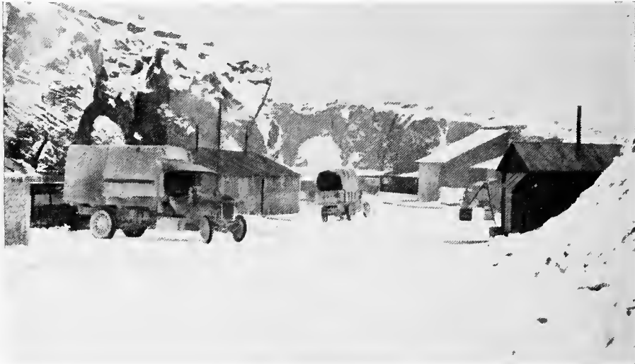
SOUTH END OF QUARRY, RATTENTOUT, SHOWING OFFICERS' QUARTERS AND HEADQUARTERS OFFICES.
