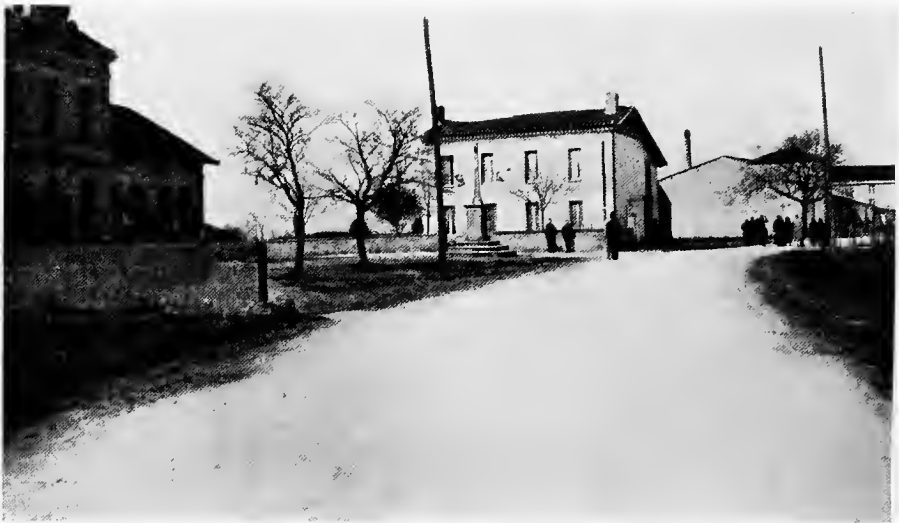
STREET SCENES IN PLUMET, WHERE COMPANY "C" WAS STATIONED
