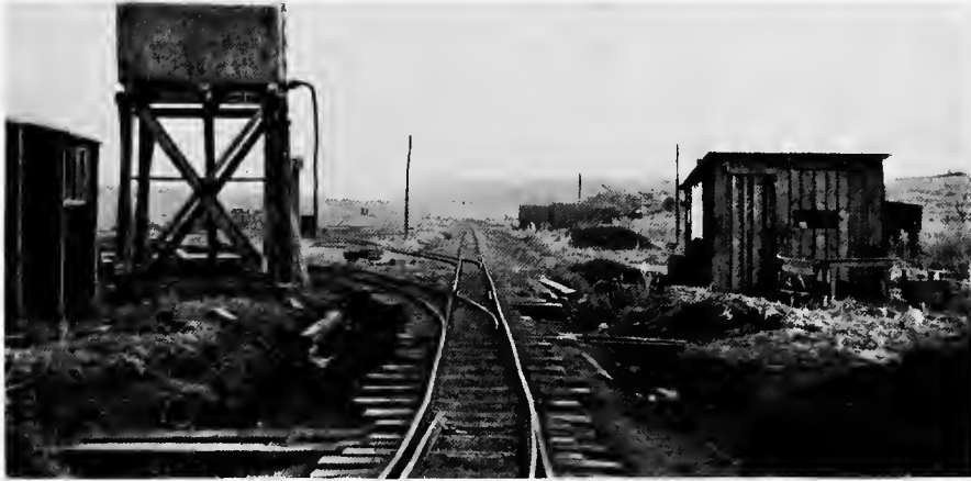
LIGHT RAILWAY YARD AT FINS
