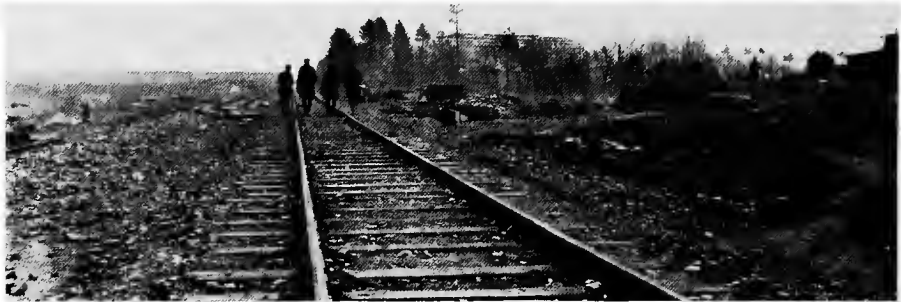
STANDARD GAUGE ROISEL-ST QUENTIN LINE THROUGH MONTIGNY, CONSTRUCTED AFTER GERMAN RETREAT OF SEPT. 1918
