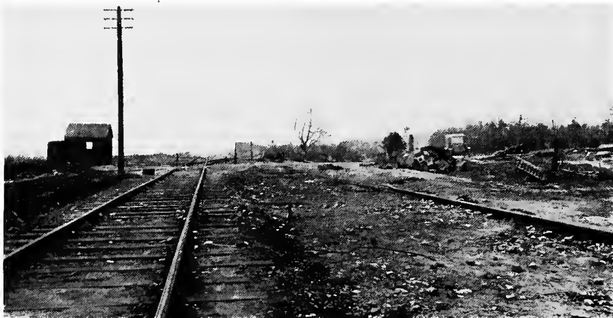
ROISEL RAILHEAD FROM THE WEST
