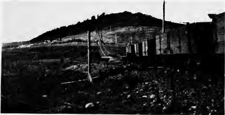
CABLE LINE BUILT BY GERMANS, VIEVILLE-SOUS-LES-COTES
