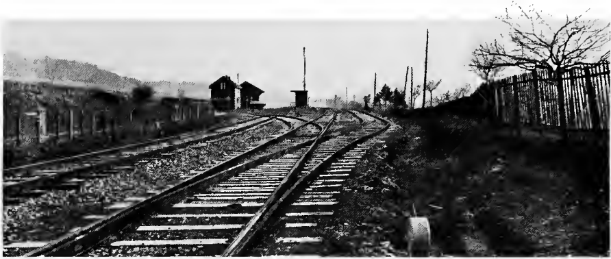
DOUBLE-TRACK CONSTRUCTION AT WIRY-AU-MONT
