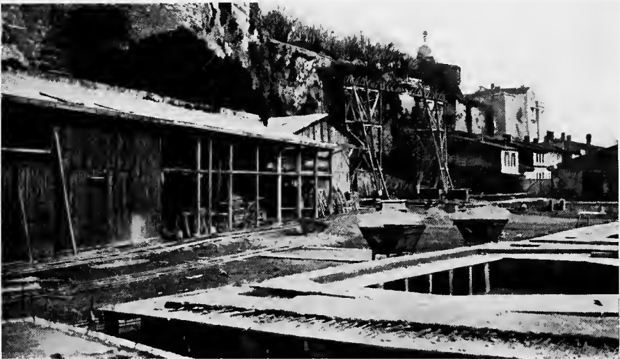
CONCRETE BOAT CONSTRUCTION, BOURG
