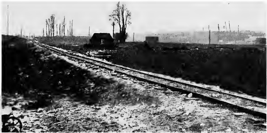
STATION C Y 5, EAST END OF ROISEL YARD
