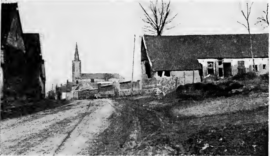
MAIN STREET THROUGH TERRAMESNIL
