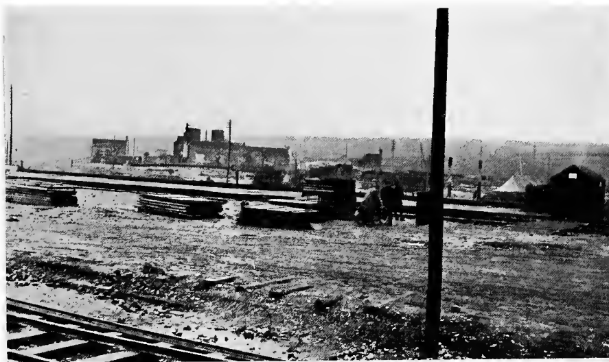
ROISEL BROAD GAUGE YARD
