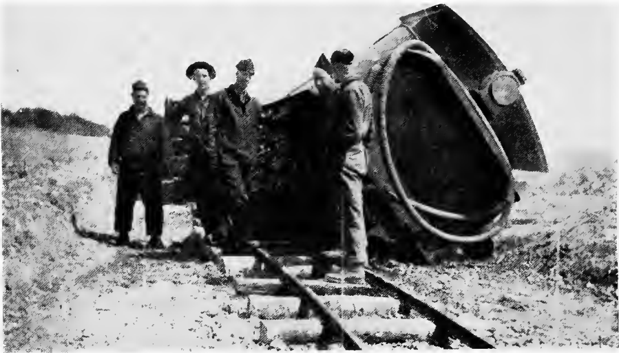
IN THE DITCH
