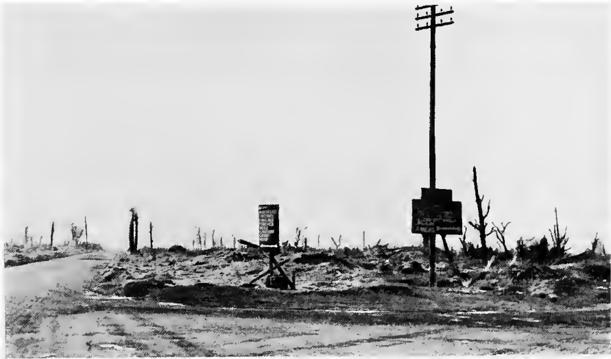
CROSSING OF AMIENS ROAD AND PERONNE-ROYE ROAD—NOTE SIGN "THIS WAS VILLERS CARBONNEL"
