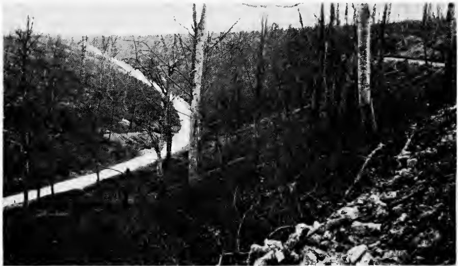
FROM MOUILLY TO THE TRENCHES, LIGHT RAILWAY ON HILLSIDE TO THE RIGHT OF THE HIGHWAY
