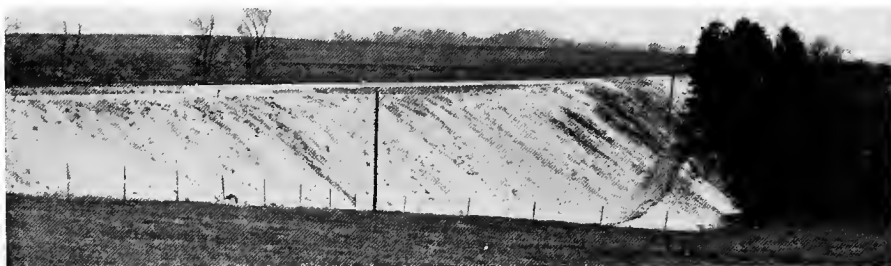
FILL JUST EAST OF WOIREL ON THE DOUBLE-TRACK CONSTRUCTION
