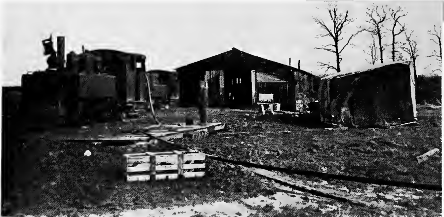
ENGINE SHED, WOINVILLE
