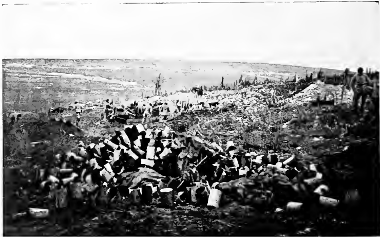
POSITION OF GERMAN BATTERY DESTROYED IN CHAUFFOUR WOOD.
