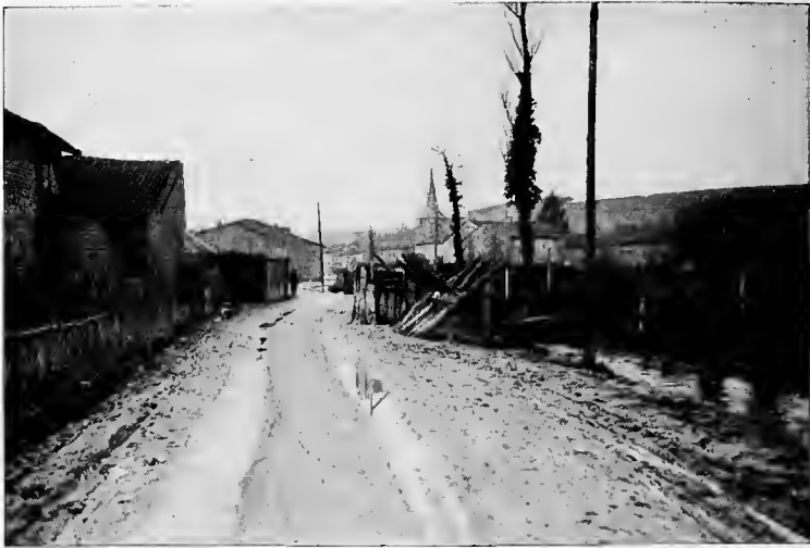
DEFENCE WORKS IN VAUX VILLAGE ( January, 1916 ).
