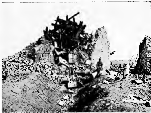
RUINS OF BRAS CHURCH, WHOSE TOWER COLLAPSED ( Photographed in April, 1917 )
