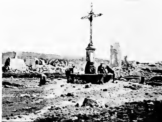
THE CROSS IN THE MIDDLE OF AVOCOURT VILLAGE IN APRIL, 1916.
