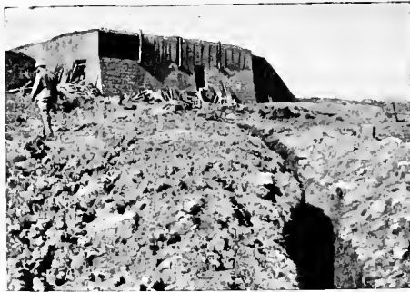
The Central Shelter having been pierced by a shell on May 6th, the Redoubt was afterwards only used as an Artillery Observation-Post. The Entrance Trench in the foreground was each day levelled by enemy shells, only to be re-made during the night.
