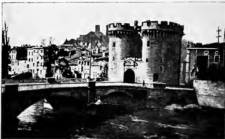
LEAVING VERDUN BY THE CHAUSSÉE GATE ( see p. 34 ).
