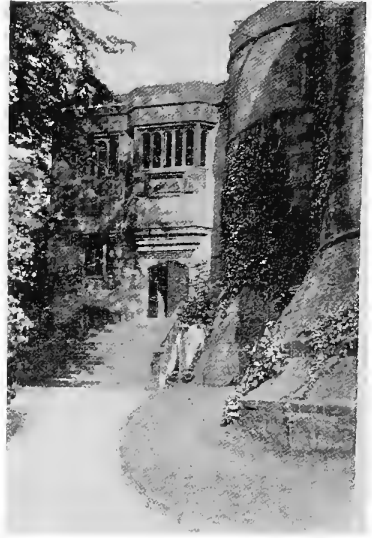
ENTRANCE TO THE CONDUIT COURT AT SKIPTON CASTLE (see page 416).
