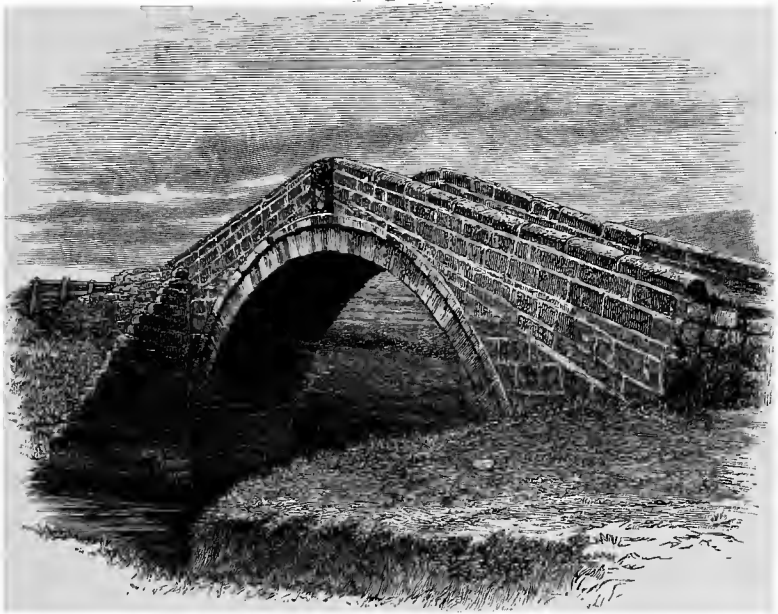
DANBY CASTLE BRIDGE. BUILT circa 1386.
