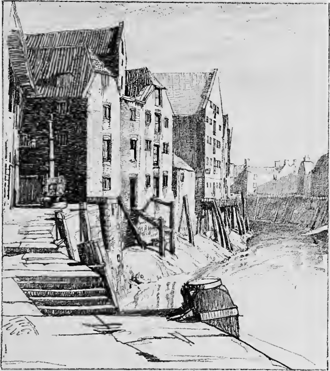
Custom House Quay, Boston.
