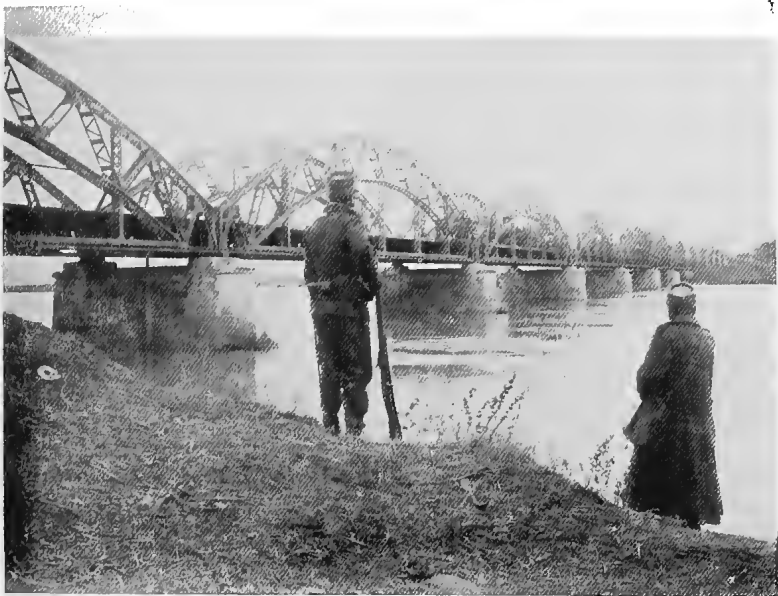
THE RAILWAY BRIDGE OVER THE VARDAR, NEAR CAVAKLI.
