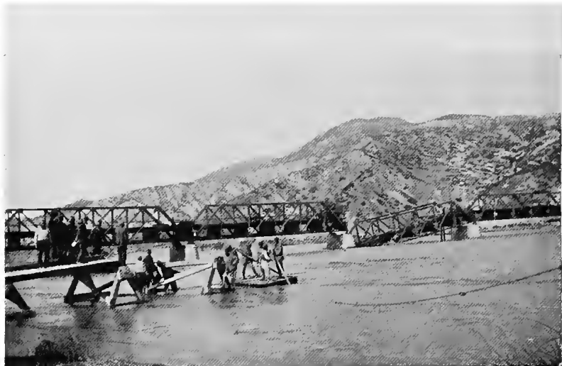
BRIDGE OVER THE STRYMON DESTROYED BY THE BULGARIANS.
