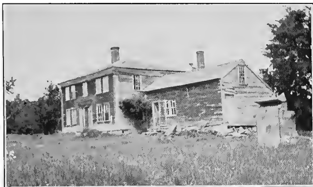
Baptist Parsonage, West Buckfield
