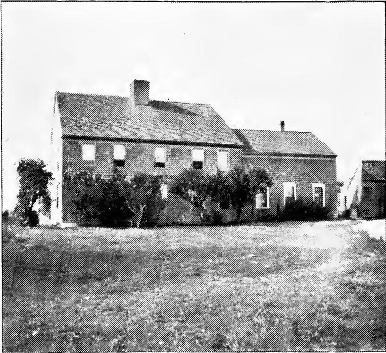
Courtesy of New Bedford Mercury.
