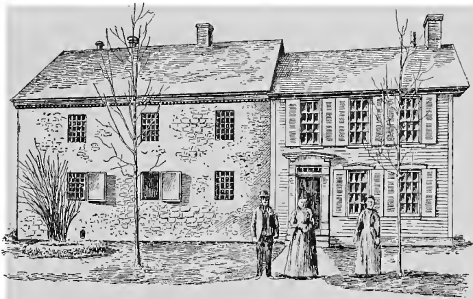
COUNTY JAIL, USED FROM 1839 TO 1894.
