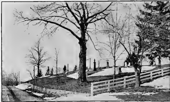
View from Northeast Corner.
