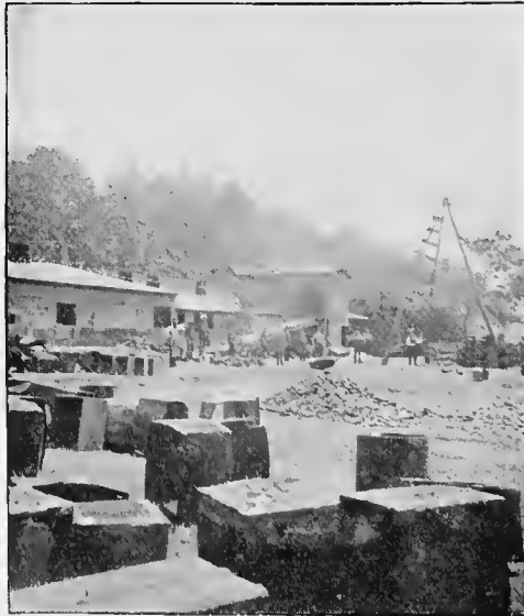
The Old Foundry Rear View.
