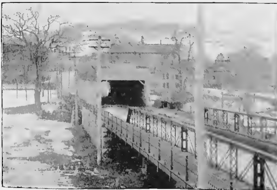
Wooden Bridge at Thomaston, Recently Demolished.
