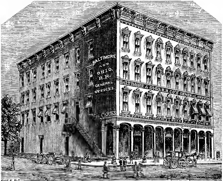
THE PARKER BUILDING,
