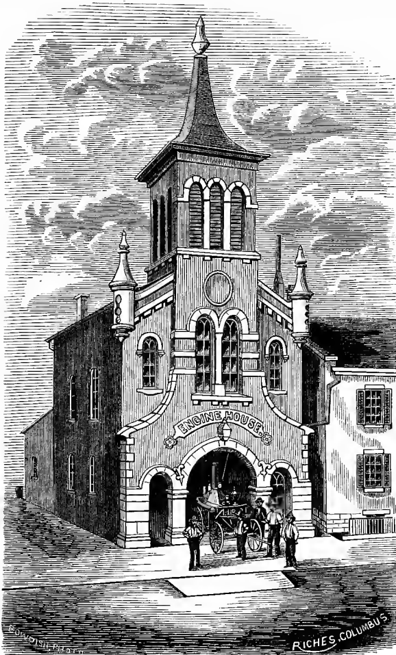
GAY STREET ENGINE HOUSE.
