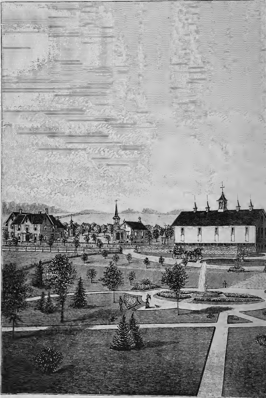
“SU RESIDENCE OF SWATARA TOWNSH
