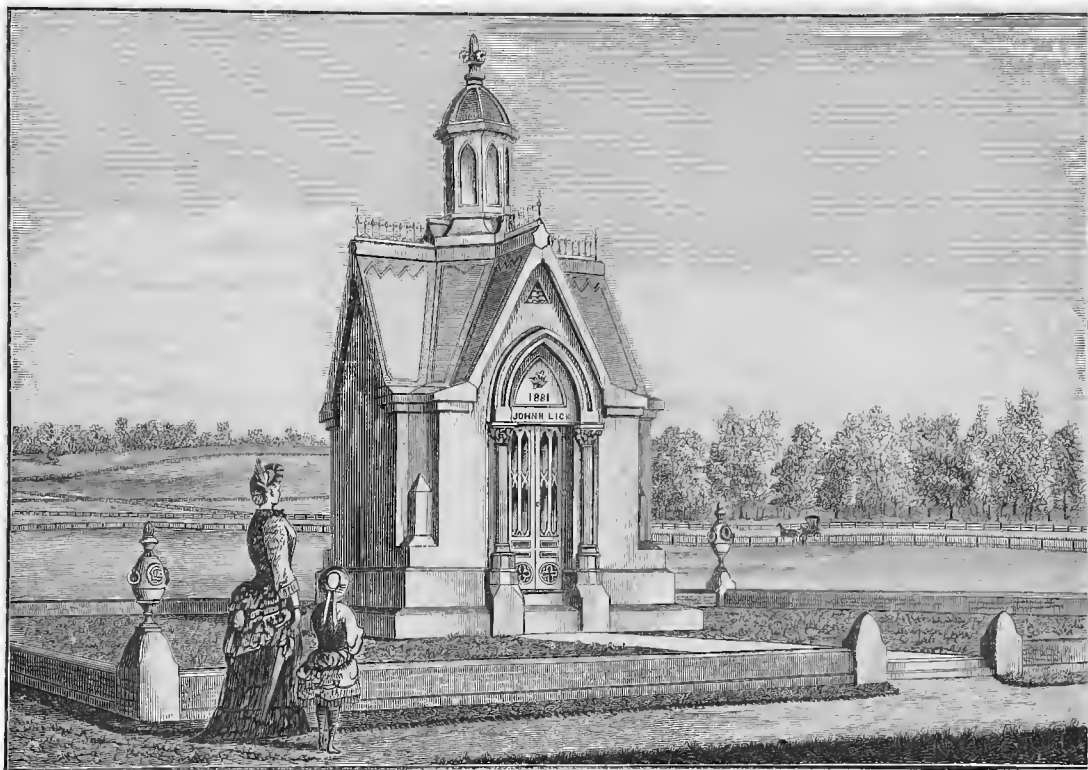
MONUMENTAL CHAPEL, FREDERICKSBURG, PA.
