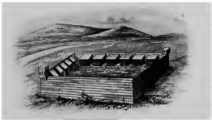
Fort Massachusetts Blockhouse, showing the garrison's barracks and the watch-towers on the exposed angles of the Fort for the discharge of the sharpshooters' rifles.
