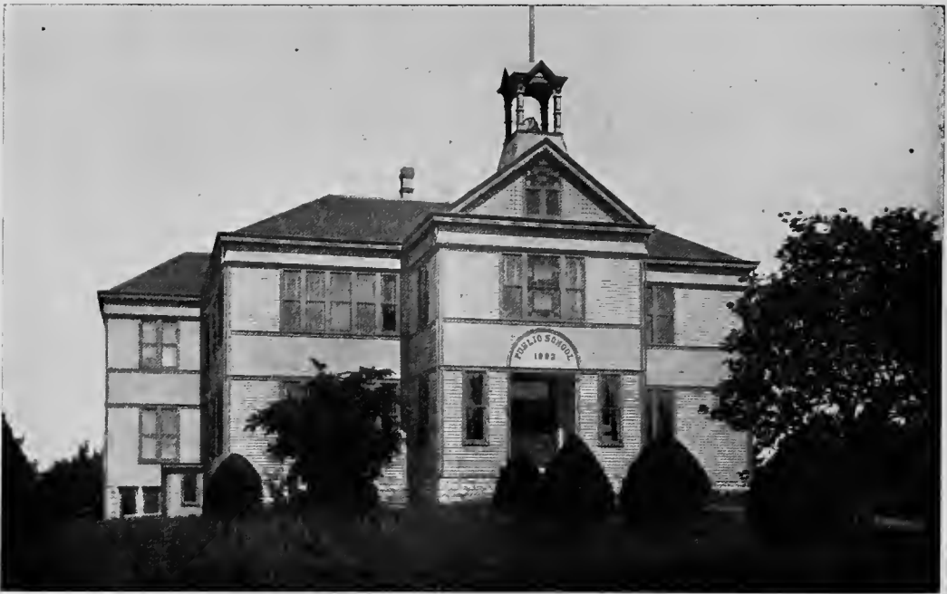
PUBLIC SCHOOL BUILDING, WETMORE, KANS.
