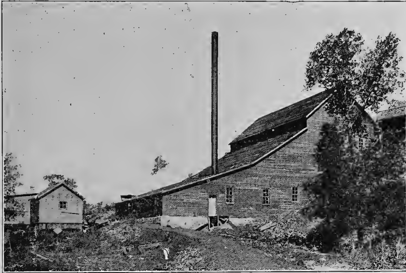
The Revenue Milling Plant.
