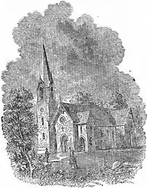
St. Peter's Church, Westchester—Erected A. D. 1855.
