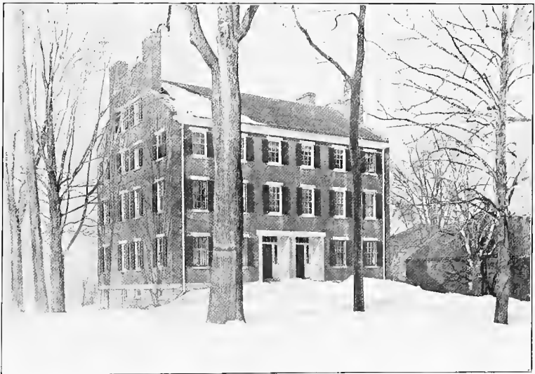
THE DOUBLE BRICK HOUSE
