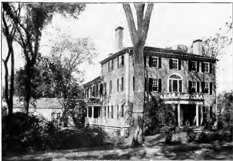
THE PRINCIPAL'S HOUSE, FORMERLY THE SAMARITAN HOUSE,
