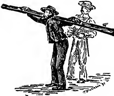
Carrying the Rail.
