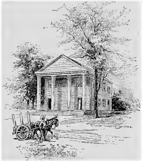
WILLIS'S CHURCH, ON THE QUAKER ROAD, NEAR GLENDALE. USED AS A CONFEDERATE HOSPITAL AFTER THE BATTLE OF MALVERN HILL.
