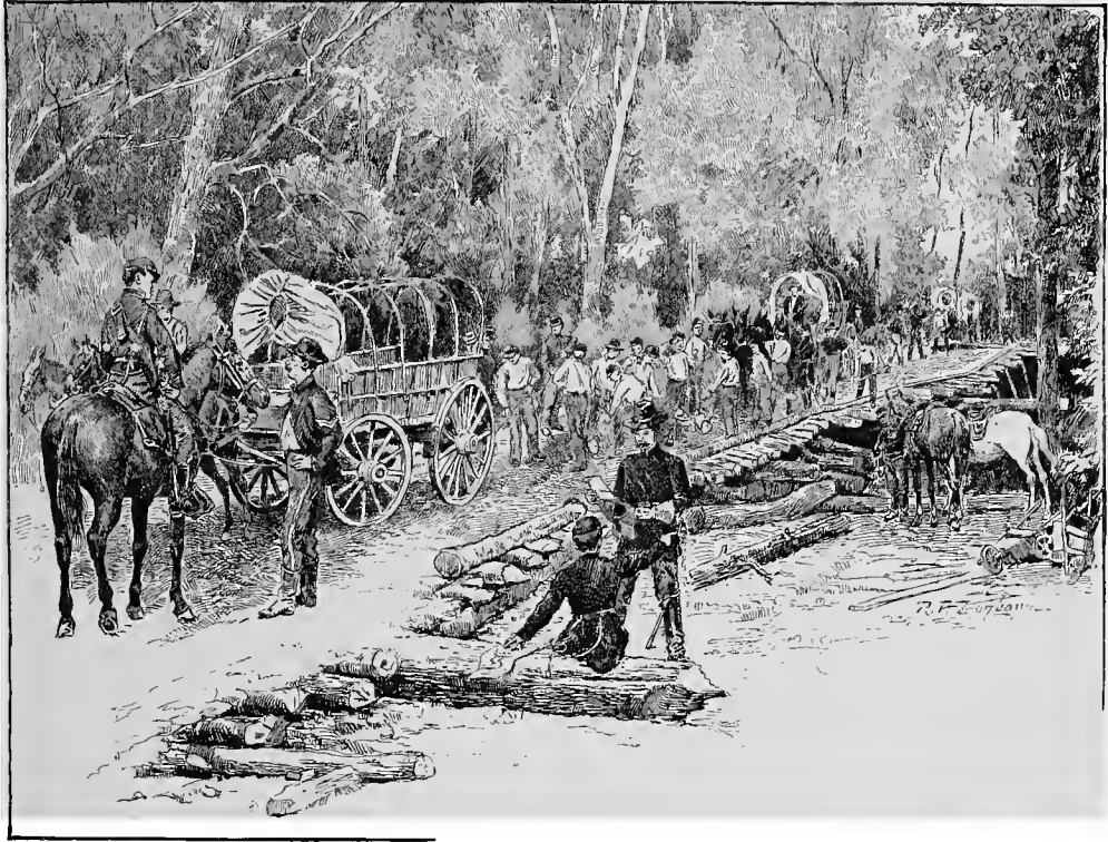
UNION TROOPS BUILDING THE CORDUROY APPROACHES TO GRAPEVINE BRIDGE. FROM A WAR-TIME PHOTOGRAPH.
