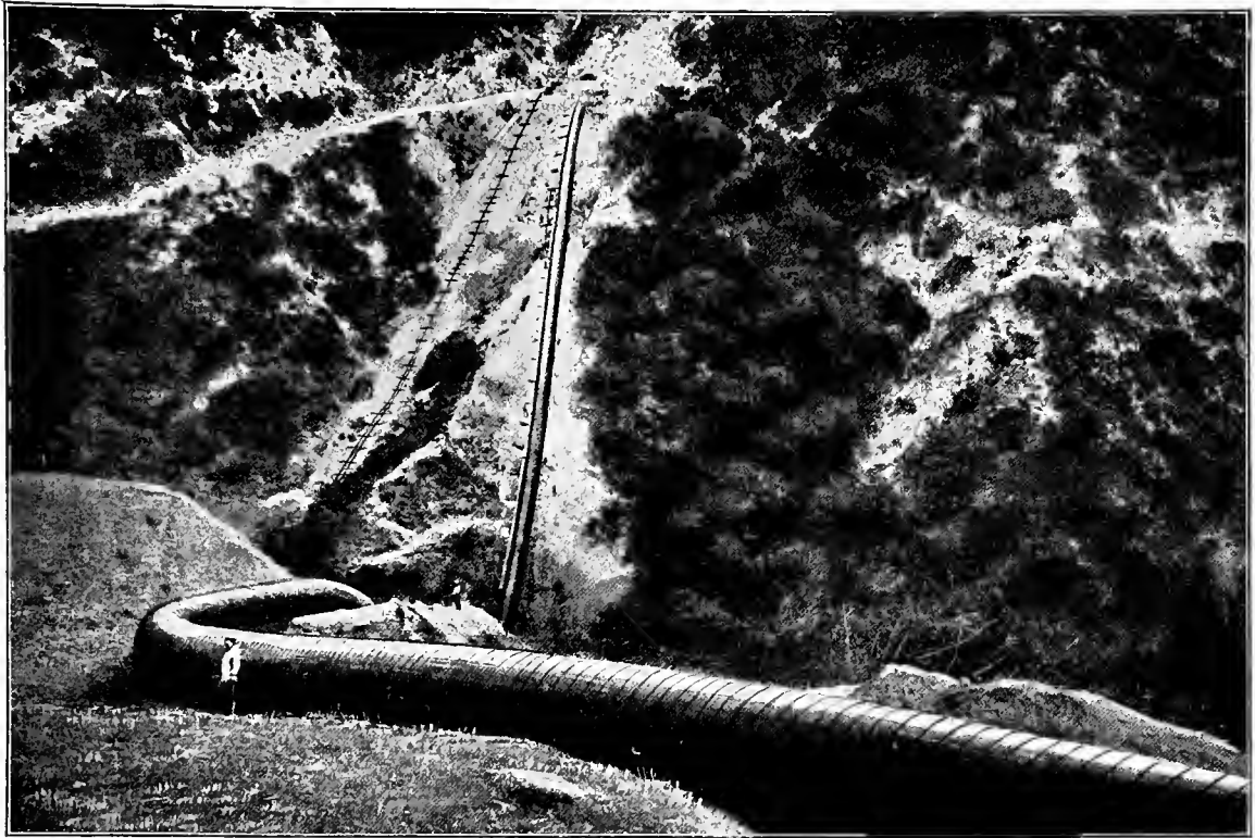
WOODEN PIPE AQUEDUCT, WITH WROUGHT-IRON RINGS.
