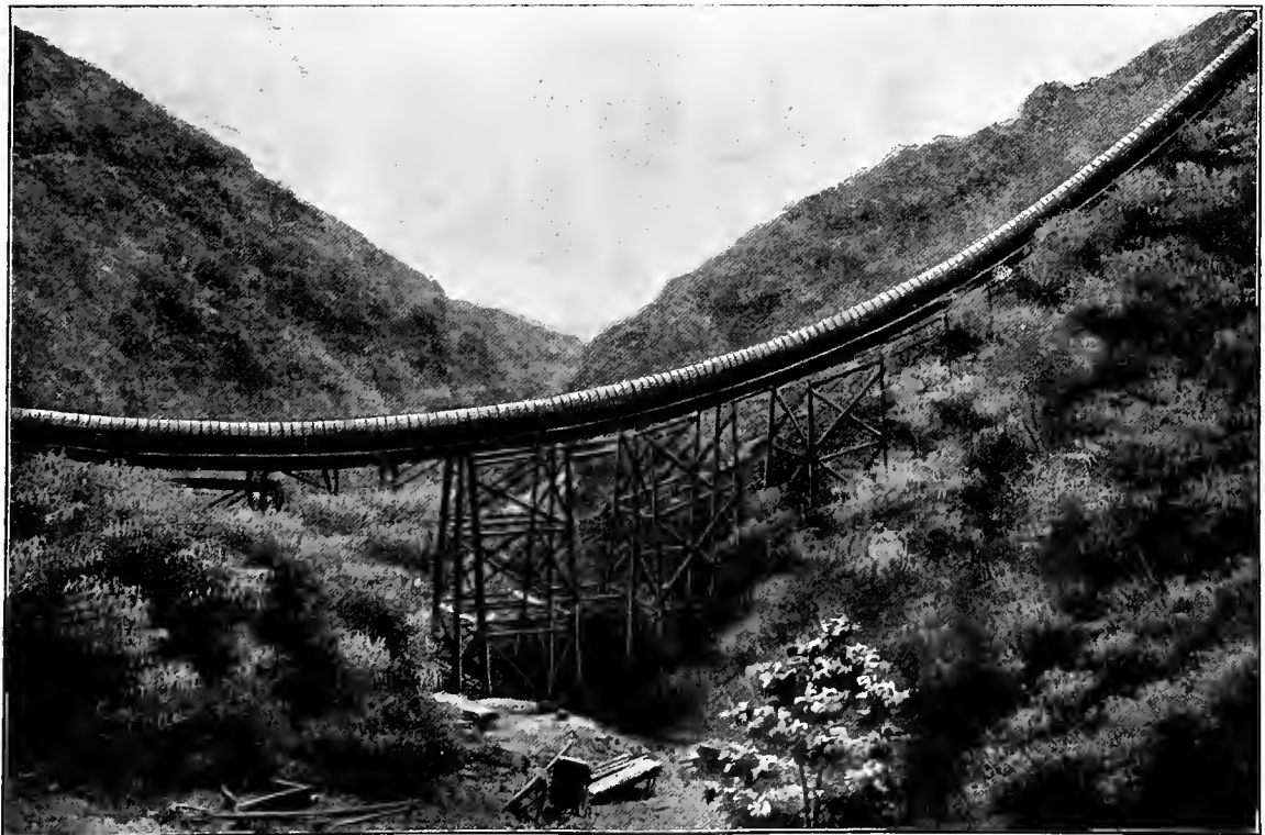
WOODEN AQUEDUCT CROSSING A VALLEY ON A TRESTLE.
