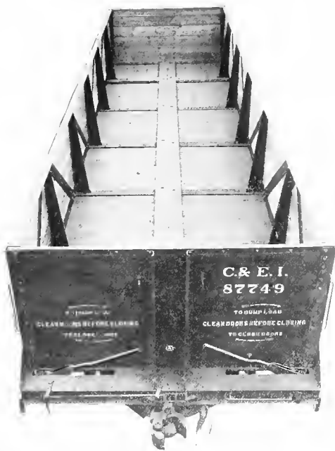
Fig. 85. National Dump Car with Drop Doors Closed.
