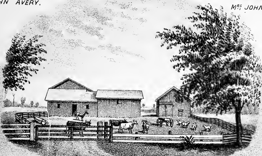
VIEW OF BARNY OPPOSITE RES.
