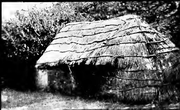
THE THREE STAGES OF MAKING LIVINGSTONE'S LAST HUT IN THE RAIN, THE LAST BEING THE ACTUAL STRUCTURE AS RECONSTRUCTED BY THE VERY MEN WHO MADE THE ORIGINAL ONE.
