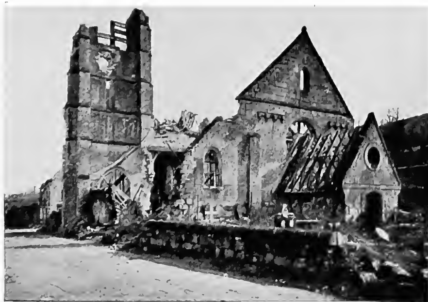
RUINED CHURCH OF ST. BANDRY.
