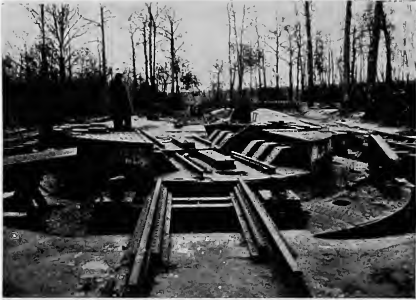
15-IN. BERTHA PLATFORM IN CHÂTELET WOOD. The road is at the back behind the trees.
