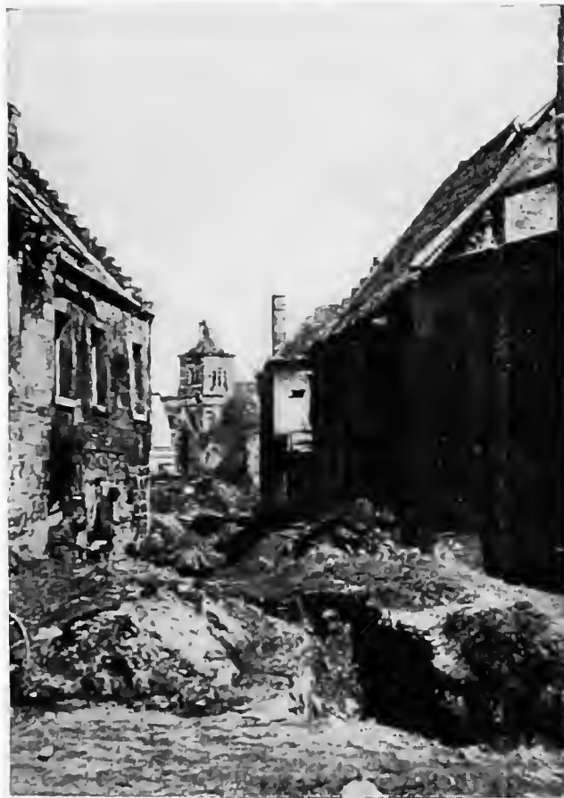
COMMUNICATING TRENCH IN ONE OF THE STREETS OF CROUY IN 1916.
