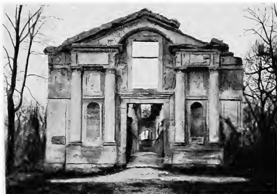
ENTRANCE TO THE GALLERY LEADING TO THE RUINS OF THE FEUDAL CASTLE OF FÈRE.
