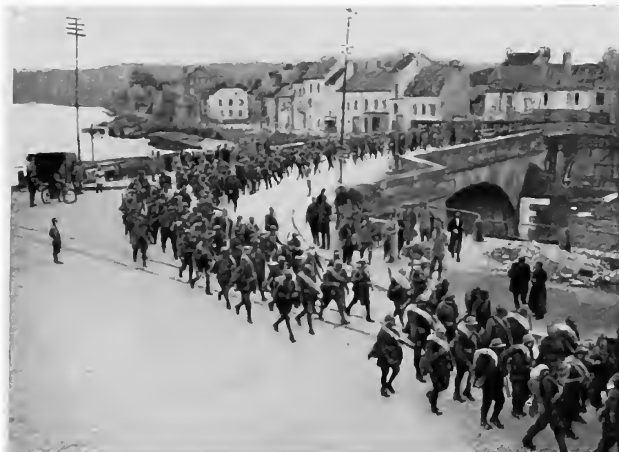
ITALIAN INFANTRY CROSSING CHÂTEAU-THIERRY BRIDGE, OF WHICH ONLY ONE ARCH REMAINS.
