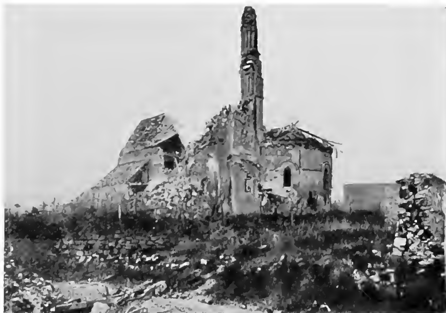
RUINED CHURCH OF OULCHY-LA-VILLE.
