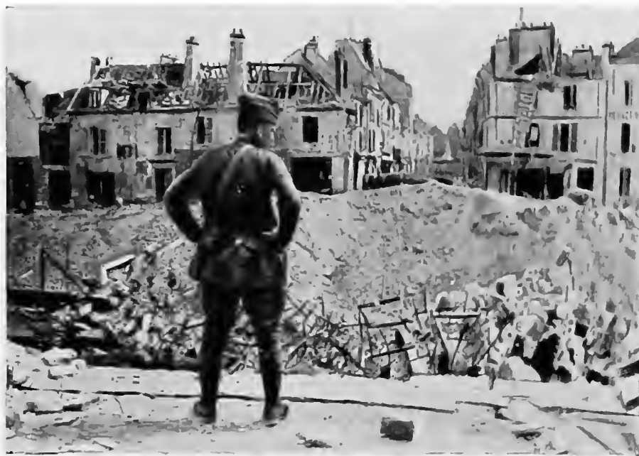
CHÂTEAU-THIERRY BRIDGE AFTER IT WAS BLOWN UP.
