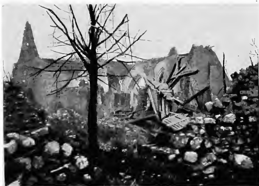
DOMMIERS CHURCH IN RUINS.
