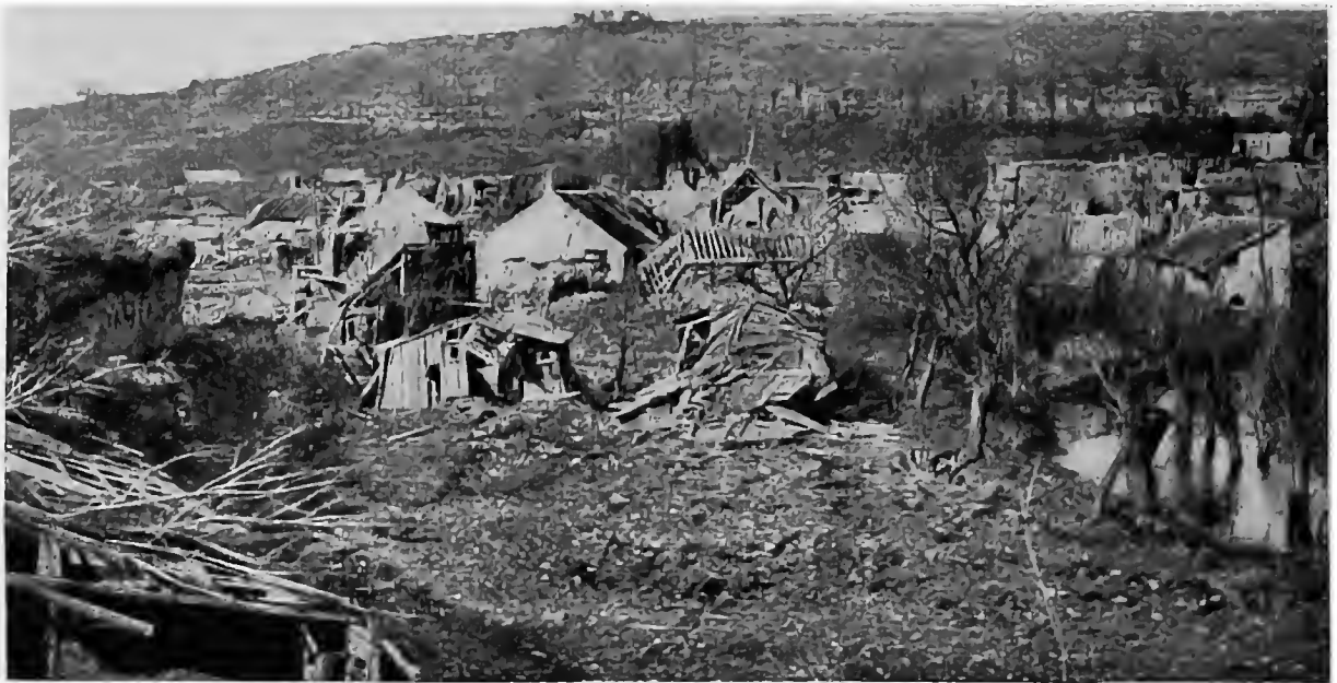
GENERAL VIEW OF BAZOCHEs.
