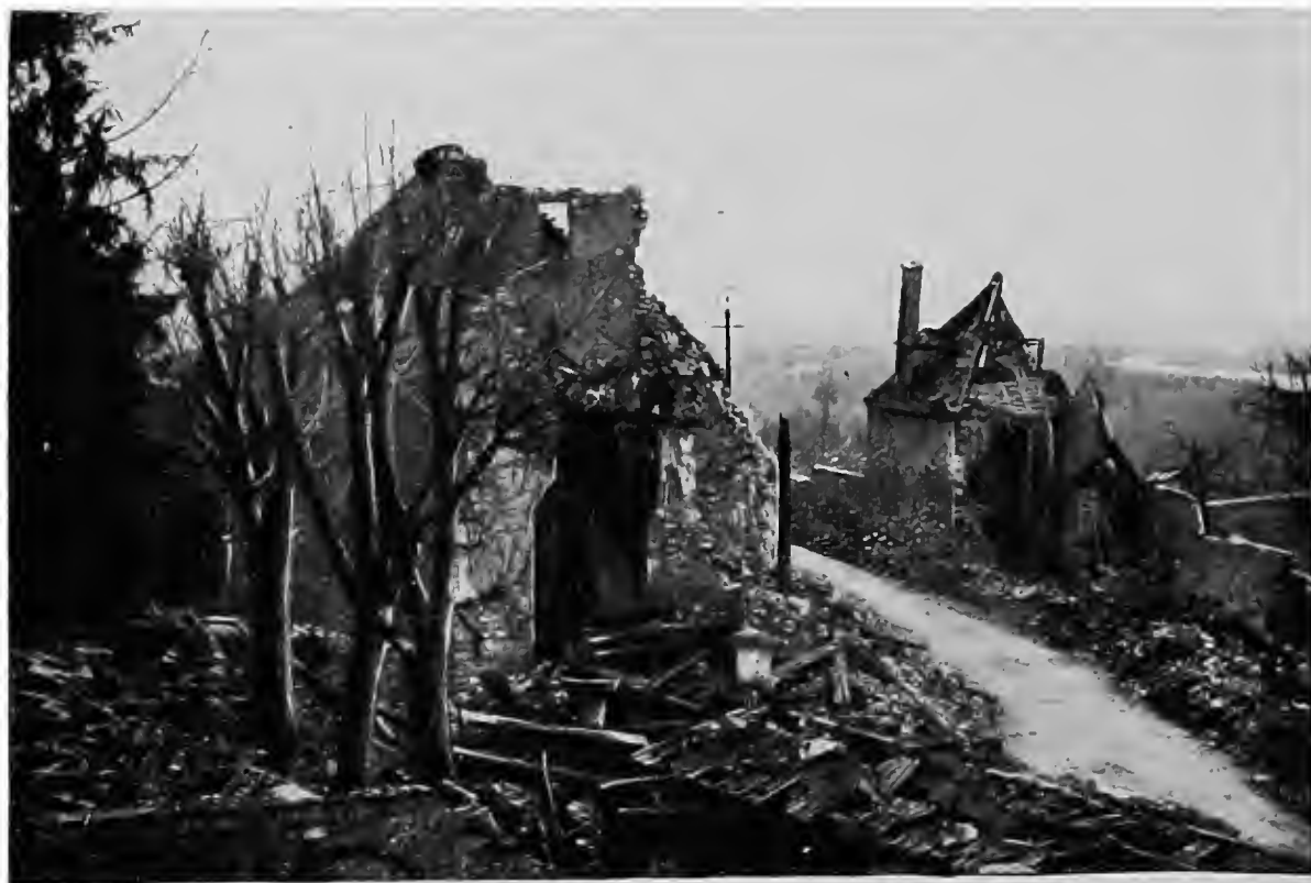
RUINED CHURCH AT MONT-ST.-PÈRE.
