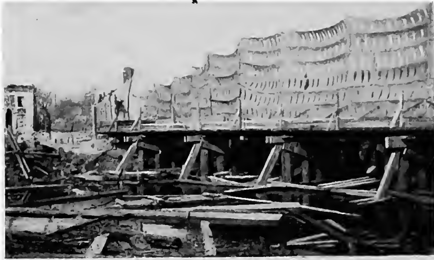
TEMPORARY BRIDGE OVER THE VESLE, "CAMOUFLAGED" DURING THE OPERATIONS.
