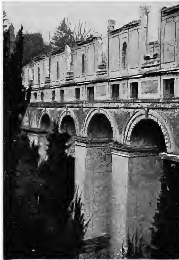
THE GREAT BRIDGE OF FÈRE CASTLE. (See below).
