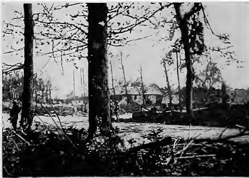
THE CROSS-ROADS AT CROIX-DE-FER, AT THE INTERSECTION OF THE N. 2 (PARIS-SOISSONS) AND THE CHAUDUN-DOMMIERS ROAD. In the background : Cravançon Farm in ruins.
