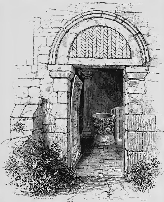
DOOR-WAY, SOUTH SIDE, LINLEY.
