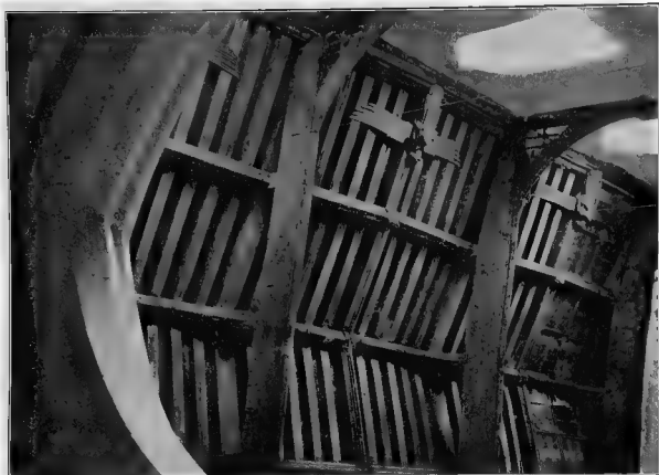
ARDLEY CHURCH : THE ROOF OF THE NAVE
