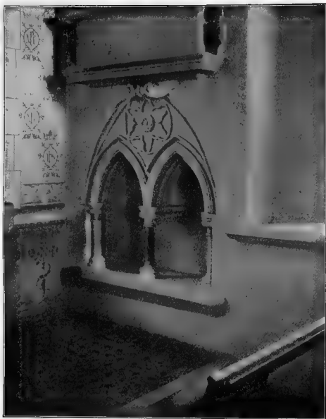
GILSTON CHURCH : PISCINA AND CREDESCENCE
