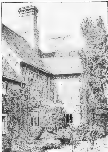
HAMMONDS FARM, PIRTON, SHOWING PORCH
