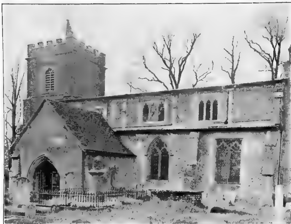
OFFLEY CHURCH FROM THE SOUTH EAST
