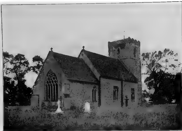
REID CHURCH FROM THE NORTH EAST
