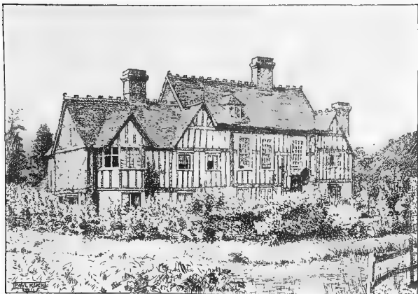
PIRTON GRANGE: EAST FRONT
