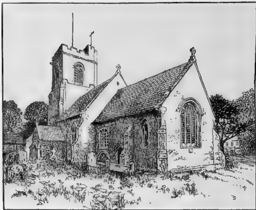
WILLIAN CHURCH FROM THE SOUTH-EAST
