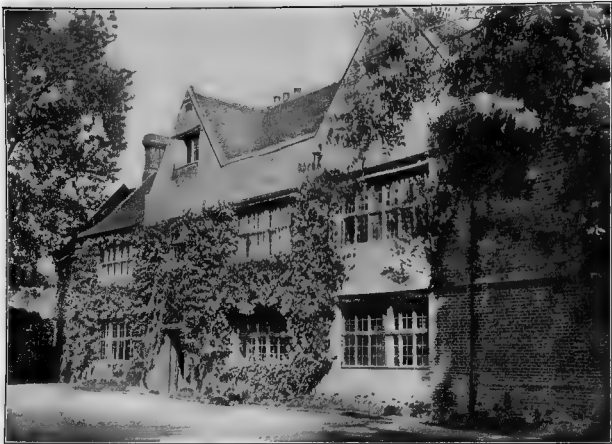
BRAUGHING: UPP HALL FROM THE WEST
