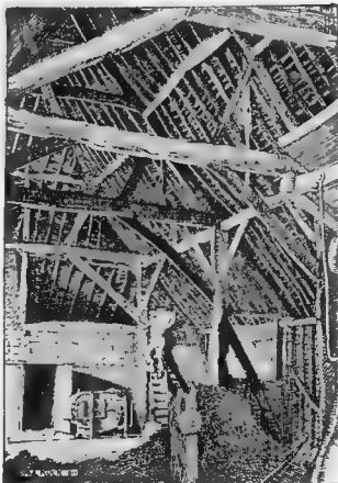
BURSTEADS : INTERIOR OF GREAT BARN
