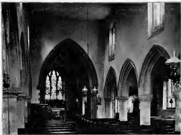
KIMPTON CHURCH : THE NAVE LOOKING EAST
