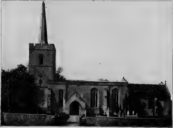
COTTERED CHURCH FROM THE SOUTH
