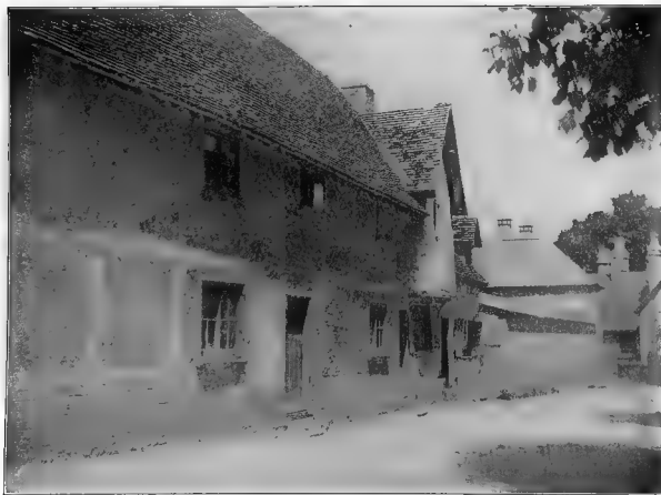
ASHWELL : OLD HOUSE NEAR CHURCH
