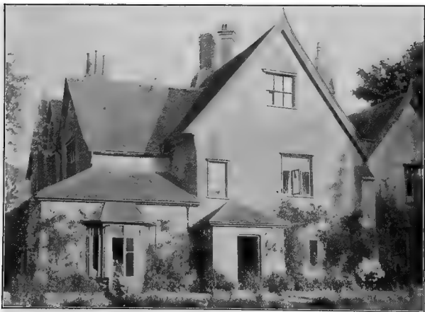
LITTLE WYMONDLEY PRIORY FROM THE NORTH-WEST
