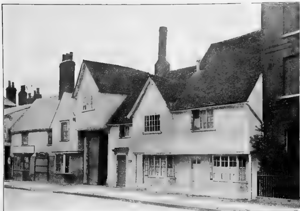
HITCHIN : OLD HOUSES IN BANCROFT
