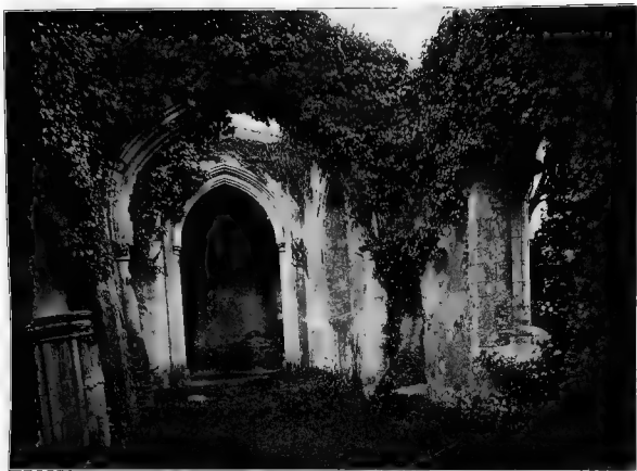
AYOT ST. LAWRENCE OLD CHURCH : REMAINS OF NORTH CHAPEL AND AISLE
