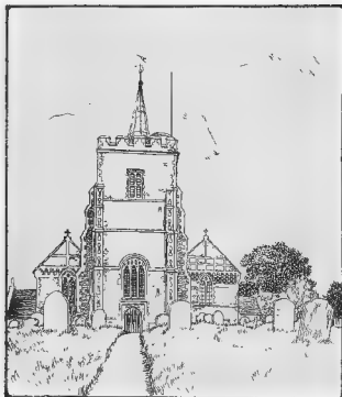
ESSENDON CHURCH: WEST TOWER
