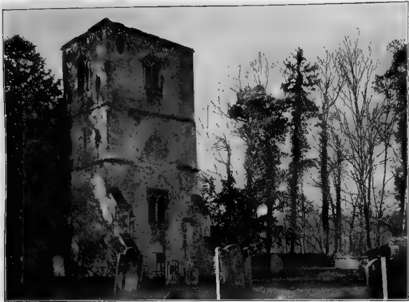
THUDRIDGE OLD CHURCH: THE TOWER
