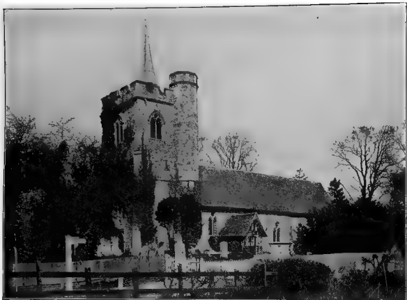
STANSTEAD ABBOTS OLD CHURCH FROM THE SOUTH WEST
