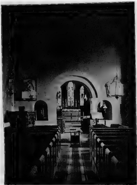
GREAT AMWELL CHURCH : THE NAVE LOOKING EAST
