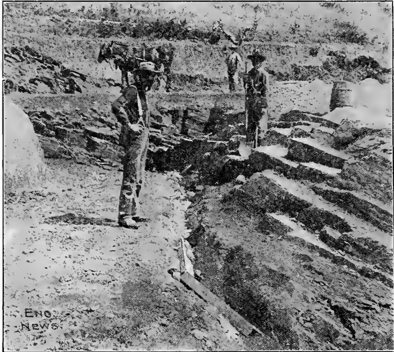
FIG. 7.—VIEW OF NORTH TRENCH, TABEAUD DAM.
