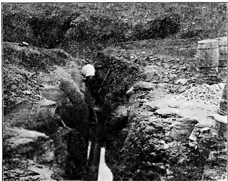
FIG. 9.—VIEW OF MAIN CENTRAL DRAIN, TABEAUD DAM.
