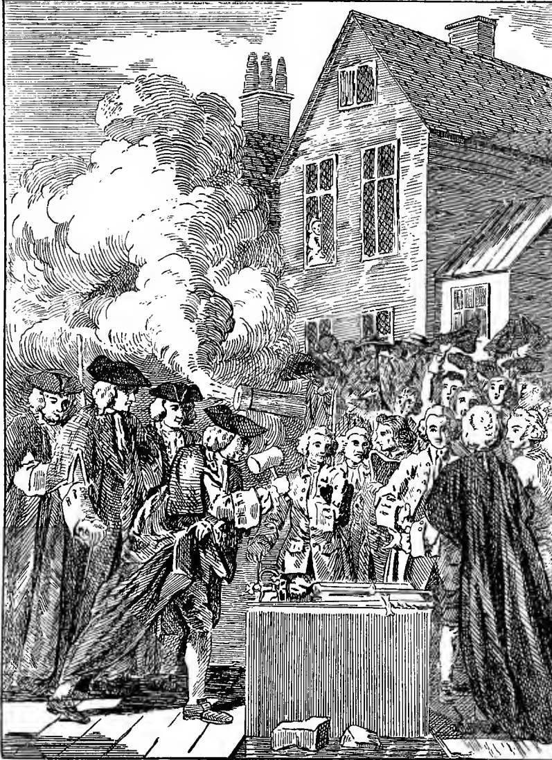
LAYING THE FOUNDATION-STONE OF BLACKFRIARS BRIDGE, 1760. From a Contemporary Print. (See page 206.)
