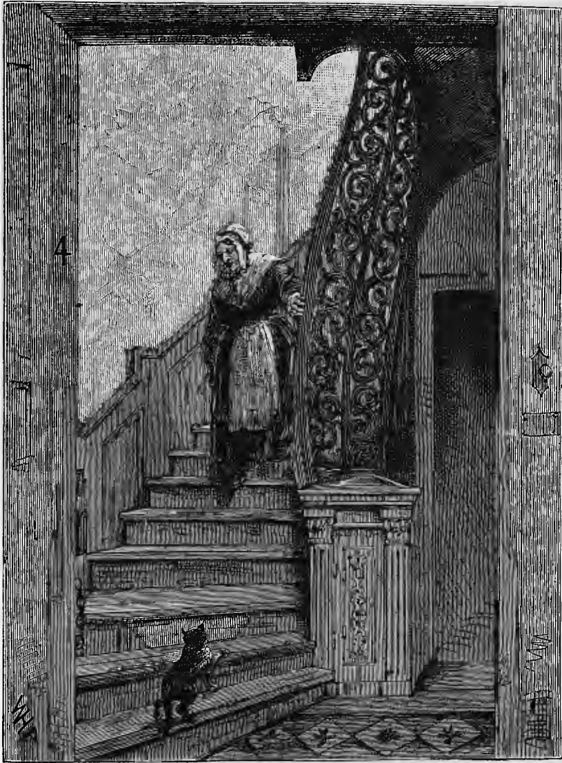
STAIRCASE IN SOUTHAMPTON HOUSE.
