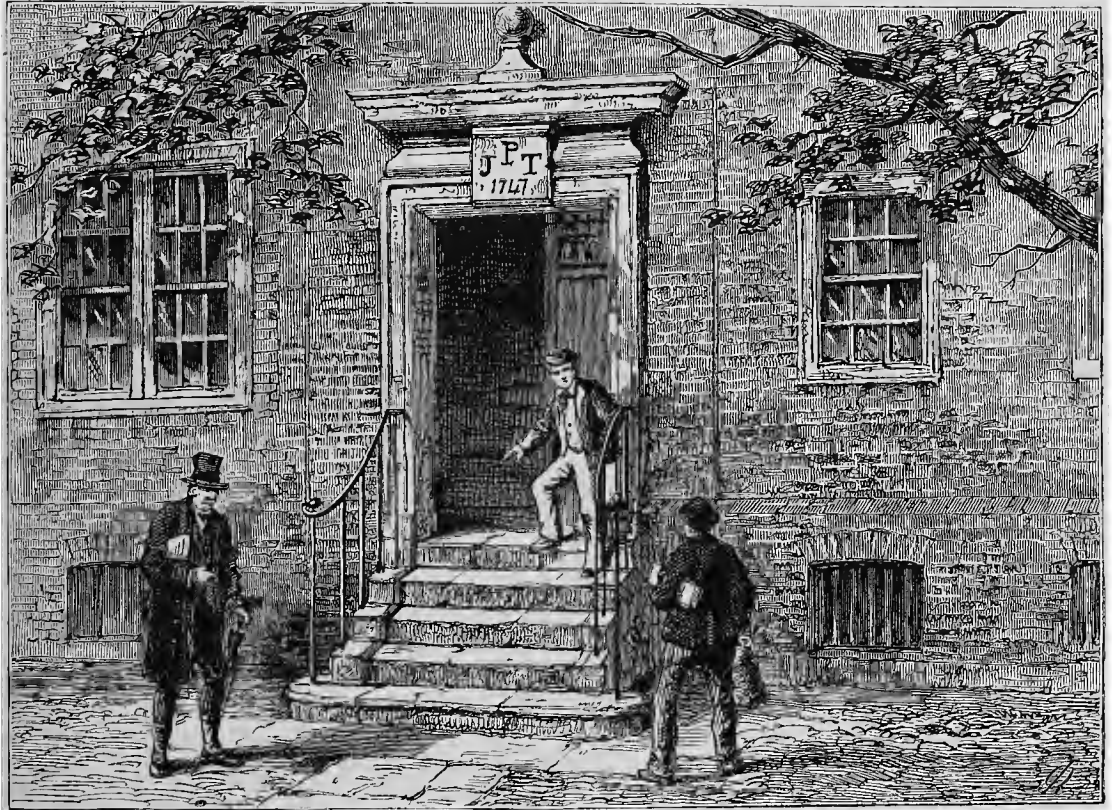
DOORWAY IN STAPLE'S INN.
