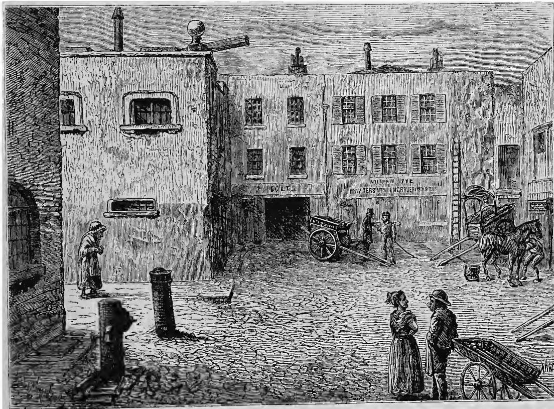
BLEEDING HEART YARD.
