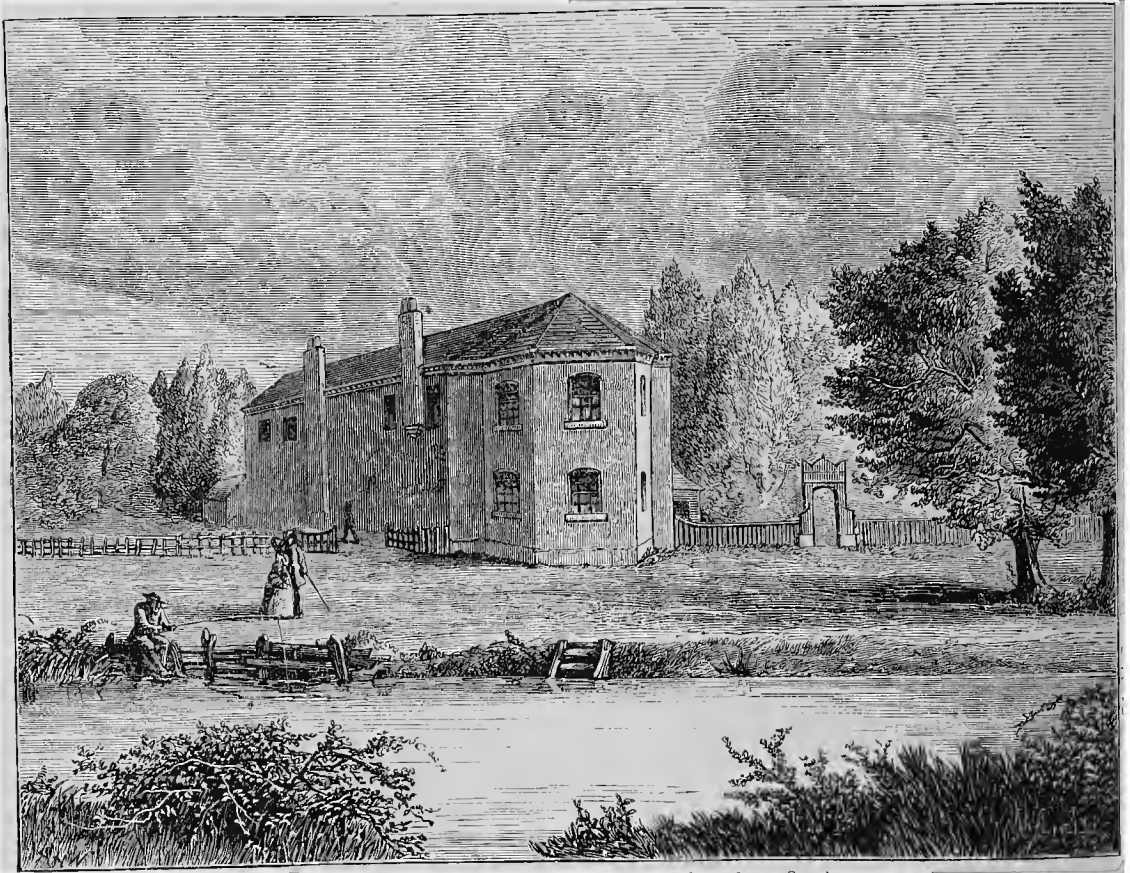
COPENHAGEN HOUSE. (From a View taken about 1800.)
