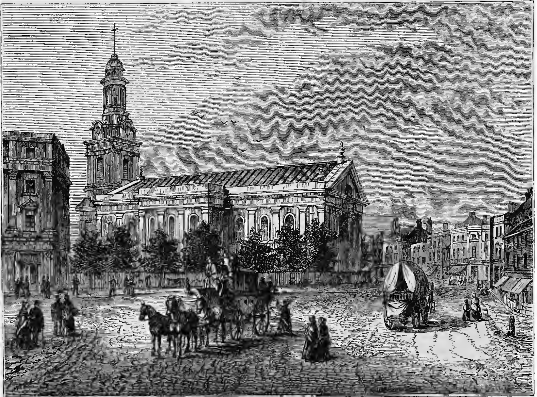
THE PARISH CHURCH, GREENWICH.
