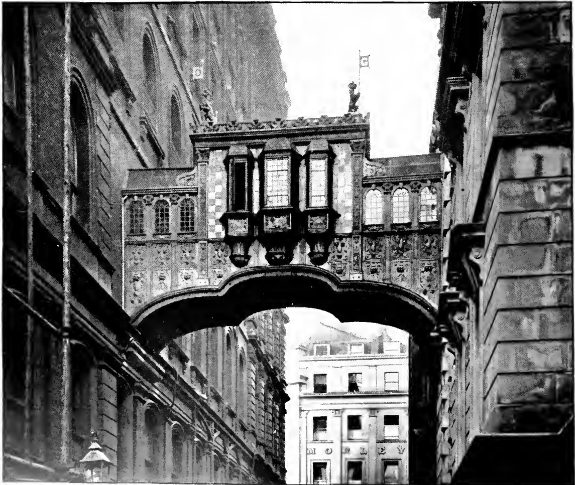
COVERED BRIDGE OF IRON, SHEATHED IN CAST LEAD, GRAND HOTEL, LONDON. Designed by WILLIAM WOODWARD, and executed by STARRIE GARDNER AND Co.
