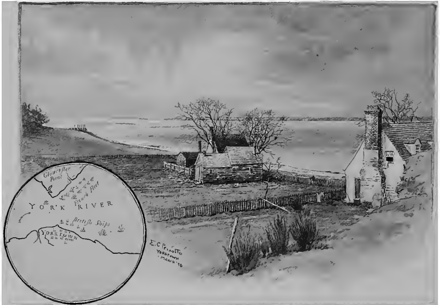
YORK RIVER, SEEN FROM THE INNER BRITISH WORKS, AND LOOKING TOWARD GLOUCESTER POINT.
