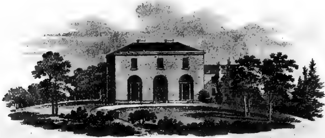
Fig. 25. Villa at Brentry Hill, shewing specimens of economy with compactness adapted to its situation, character, and uses.
