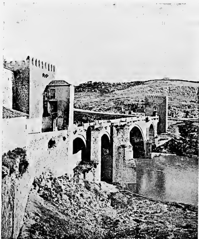
ST. MARTIN'S BRIDGE
