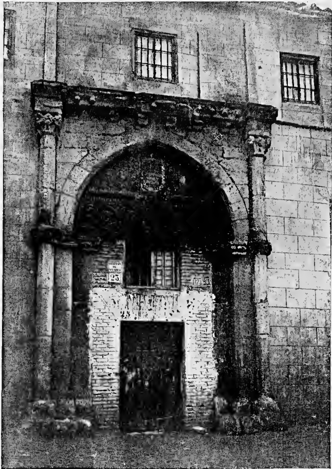
DOORWAY OF THE PALACE OF THE MARTINEZ
