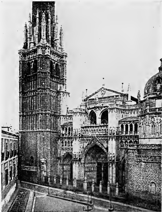
PRINCIPAL FAÇADE OF THE CATHEDRAL AND TOWER
