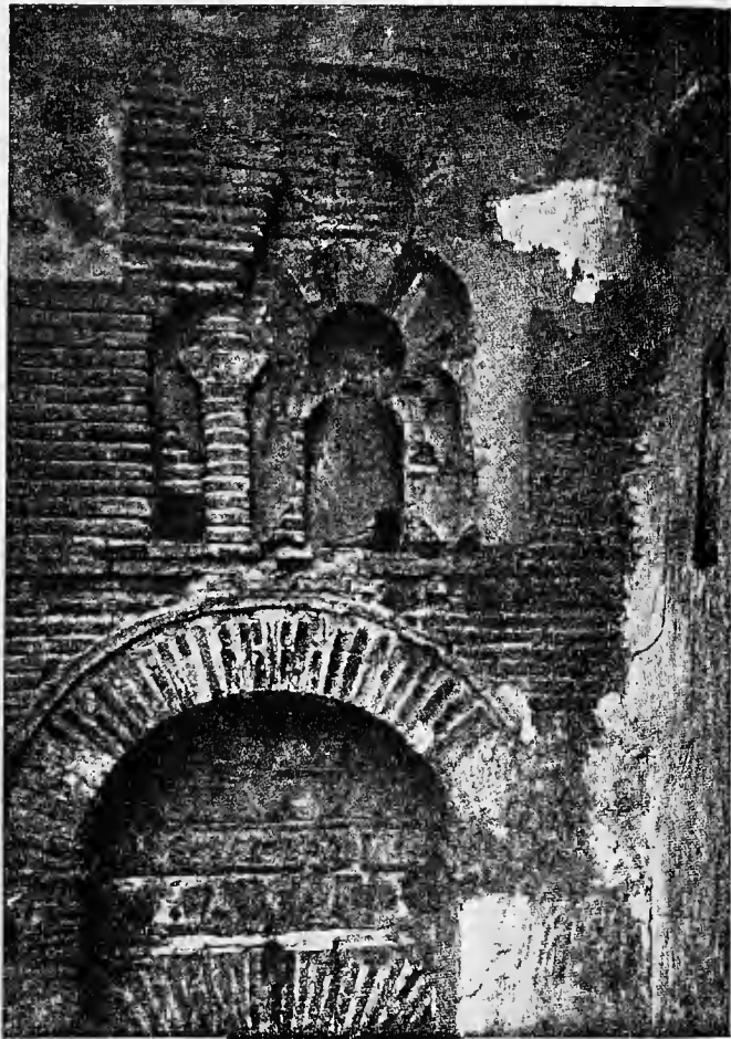
THE MOSQUE OF BIB-AL-MARDÓM, HORSE-SHOE ARCH AND REMAINS OF THE DADO OF LITTLE ARCHES AND WINDOWS IN THE NORTH-EAST FAÇADE (LEFT SIDE)
