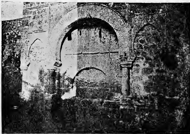
DETAIL OF THE PRINCIPAL FAÇADE OF THE OLD GATE OF VISAGRA
