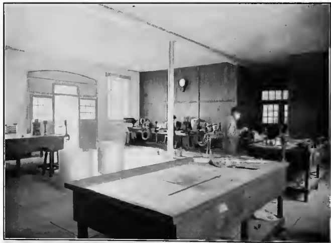
A PARTIAL VIEW OF THE TIN SHOP
