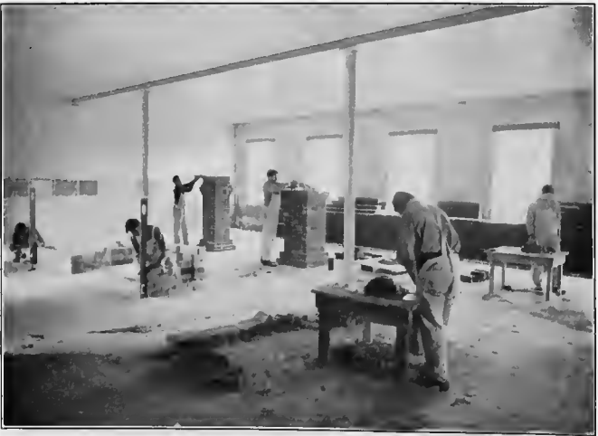
MASONRY DEPARTMENT—A LESSON IN BRICKLAYING
