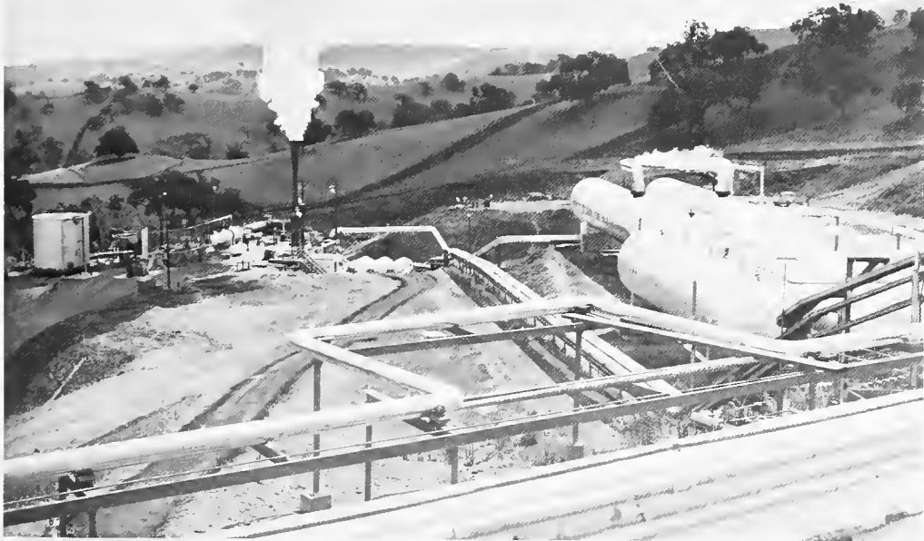
CSD's Semi-freejet Facility at Coyote Center
