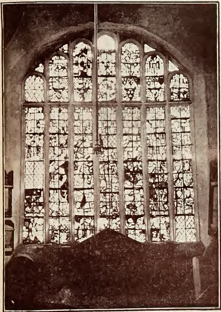
EAST WINDOW BEFORE RESTORATION, 1870.
