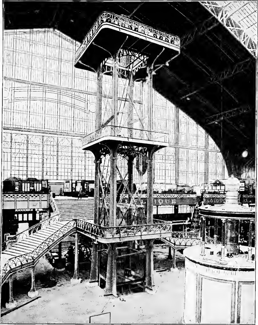
INTERIOR VIEW OF MACHINERY HALL.
