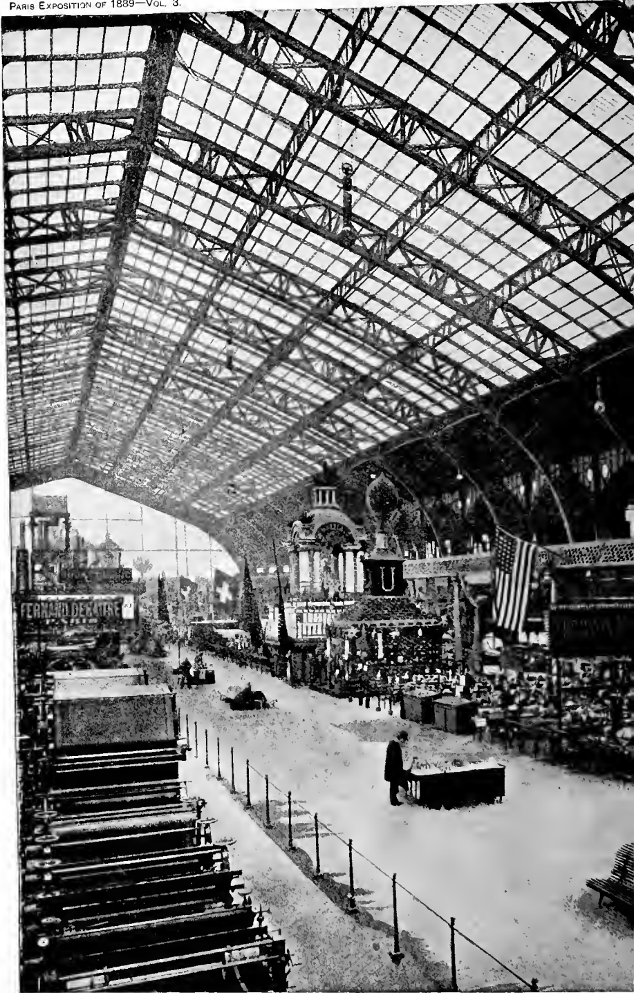
VIEW OF INTERIOR OF MACHINERY
