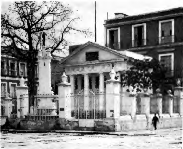
TEMPLE MONUMENT, ERECTED AT SITE OF FIRST MASS SAID IN HAVANA
