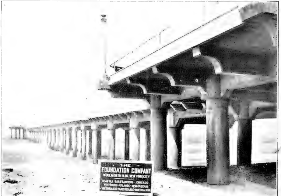
The Municipal Pier at Manhattan Beach, California. View showing Structure.
