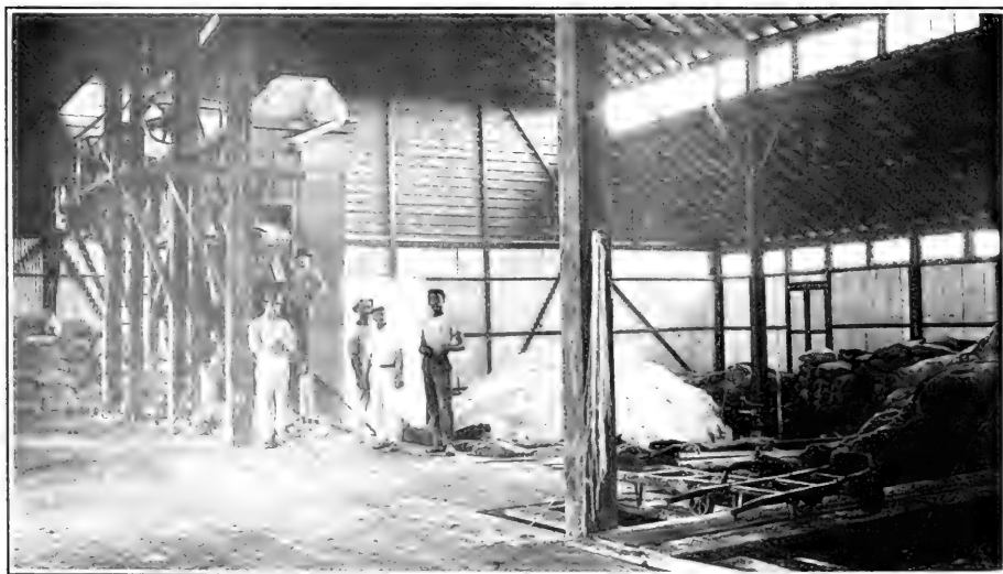
Interior View of Factory
