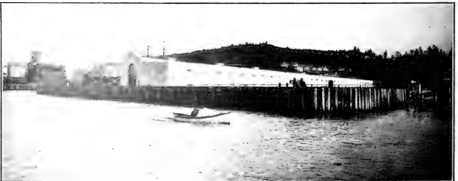
The new Astoria Pier built by The Foundation Company
