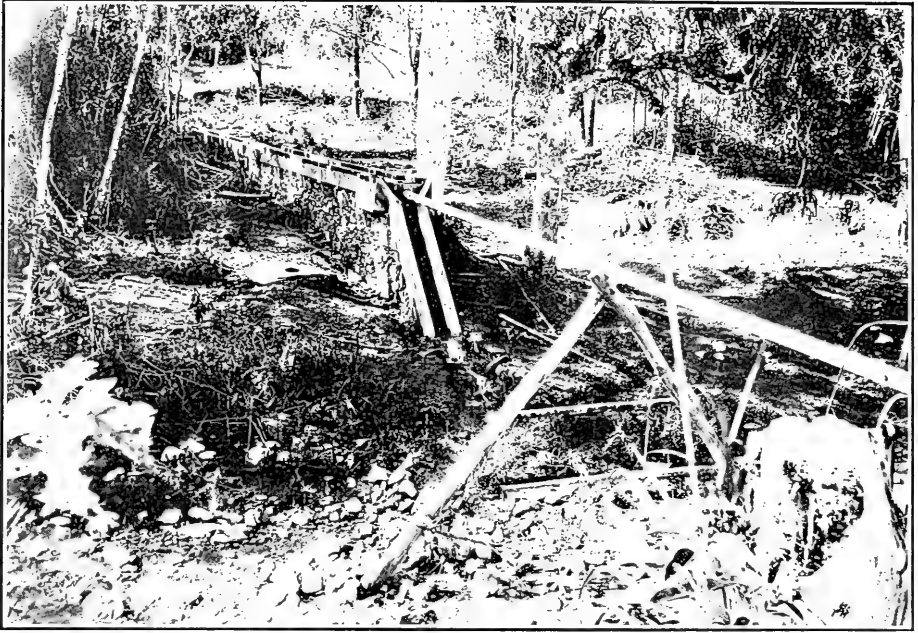
Part of Water Supply Installation, Finca Morena, Pinar del Rio Province.
