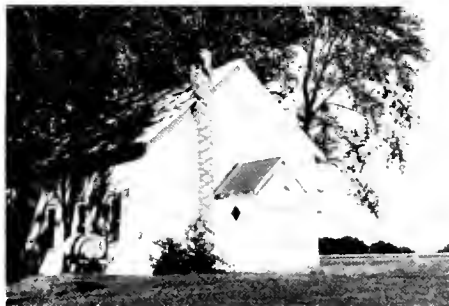
Washington Church, Crooked Creek Township
