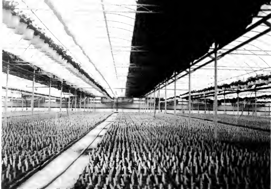
View of greenhouse showing energy saving blanket in partially closed position.
