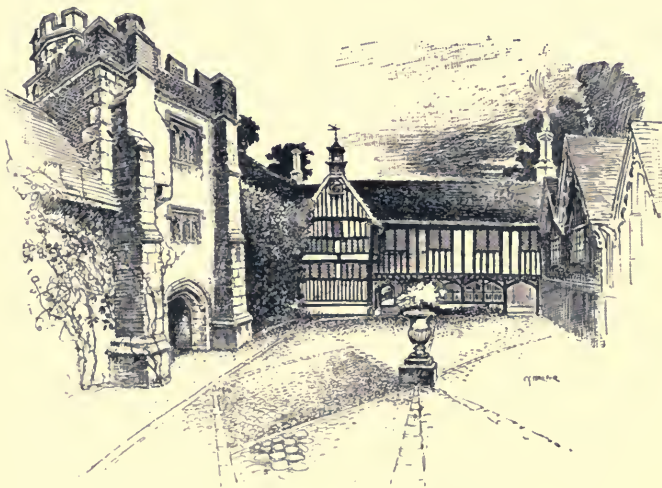
THE COURTYARD, IGHITHAM MOTE.
