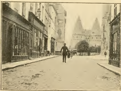
STREET SCENE, BEAUVAIS, FRANCE.
