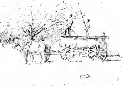
2379. Power sprayer, using steam.
