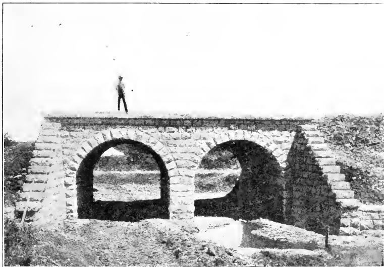
Fig. 77. Double Arch Culvert, 14 by 5½-Foot.
