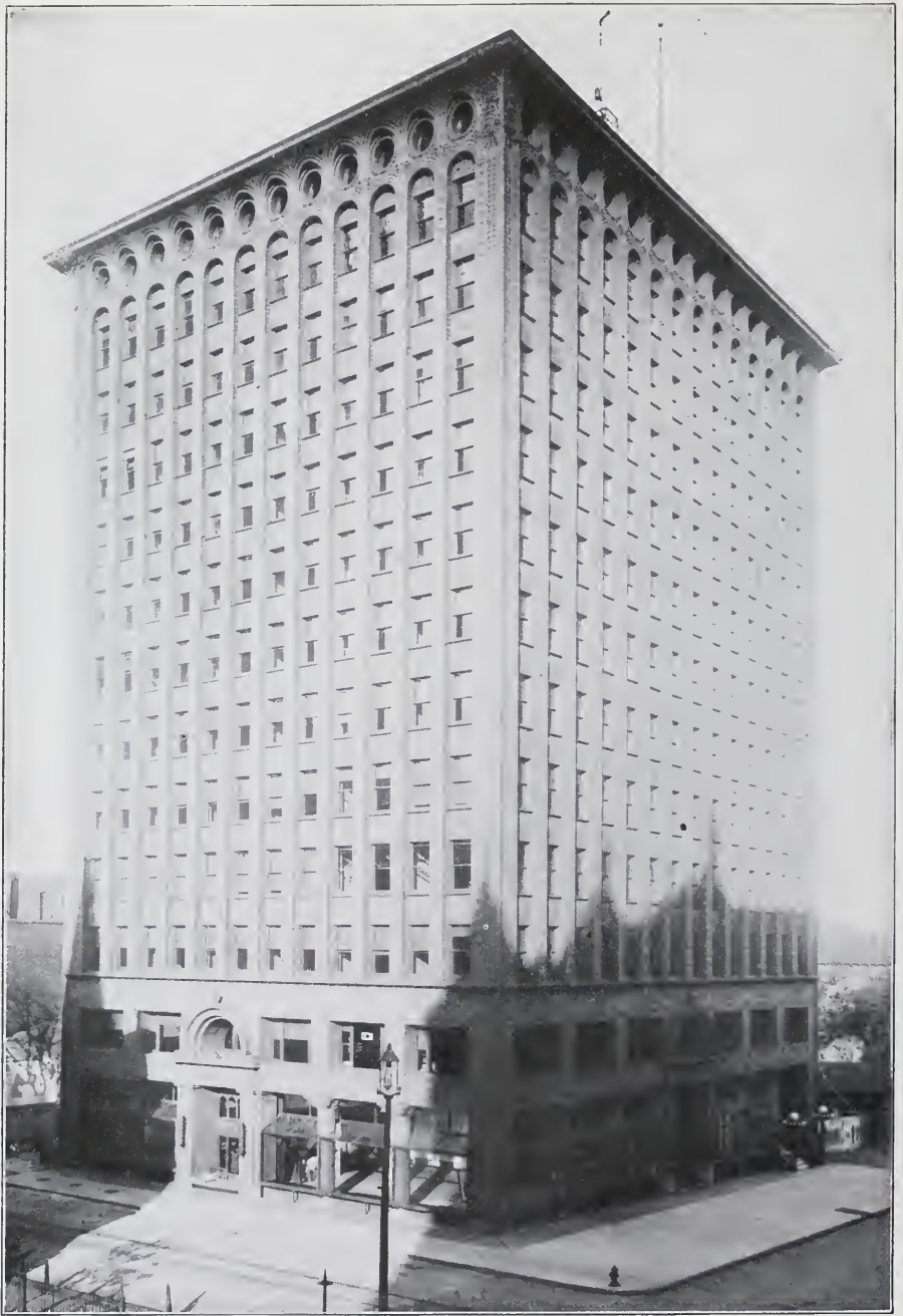
THE PRUDENTIAL BUILDING One of Buffalo's Best Office Buildings
